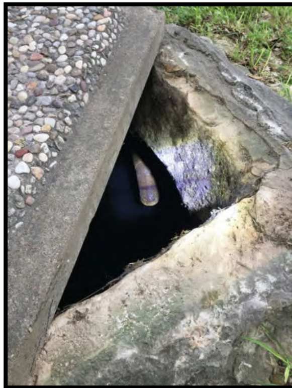
Feature S-2: Septic tank manhole near primary residence.
