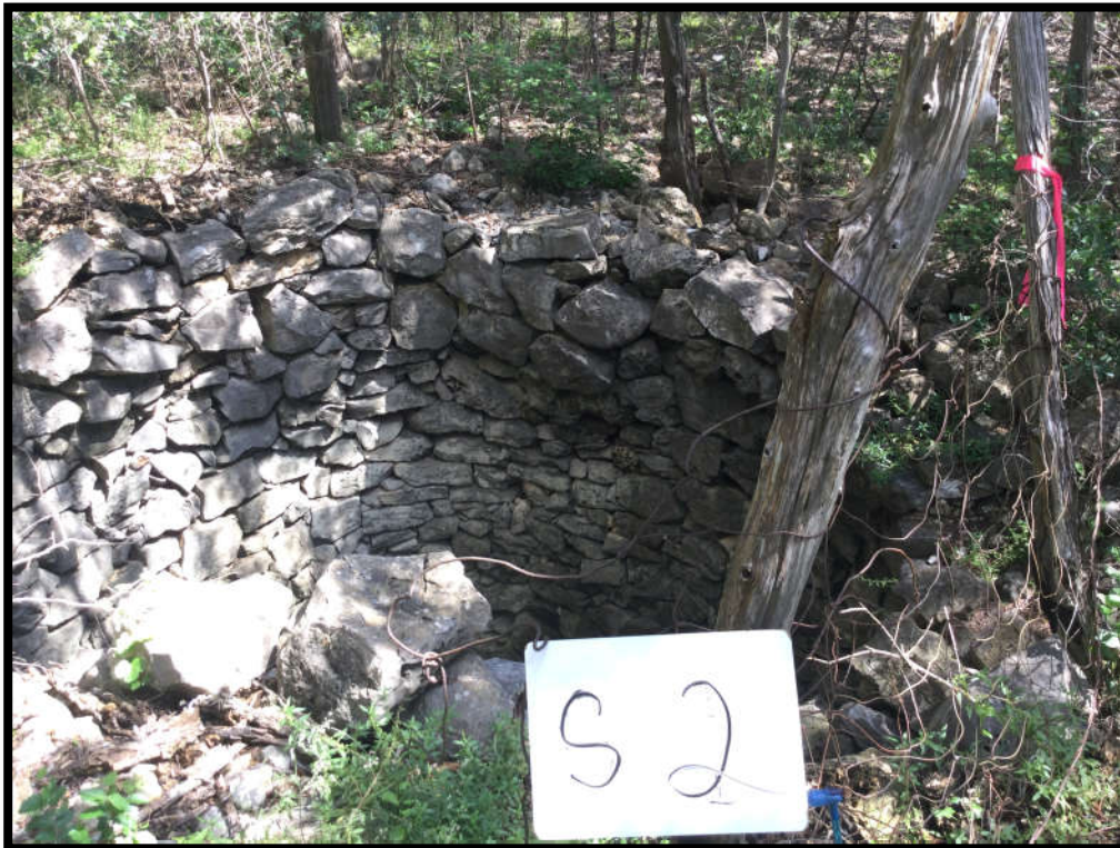
S-2: Old rock-lined, hand-dug well.
