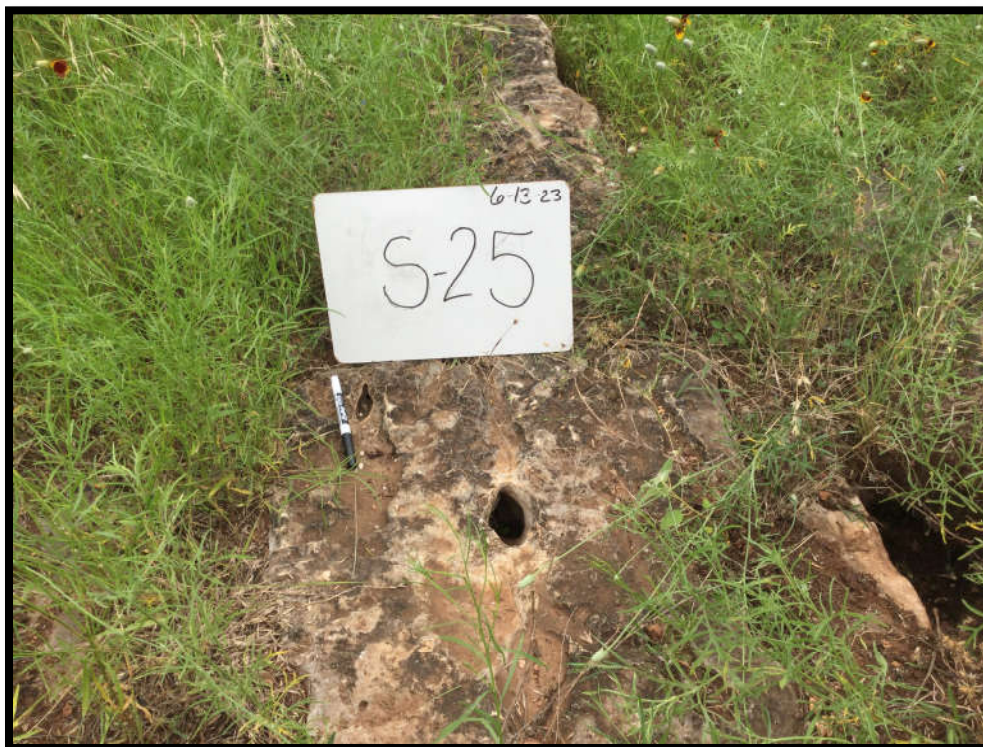
S-25: Solution cavity located on the central part of the Site.
