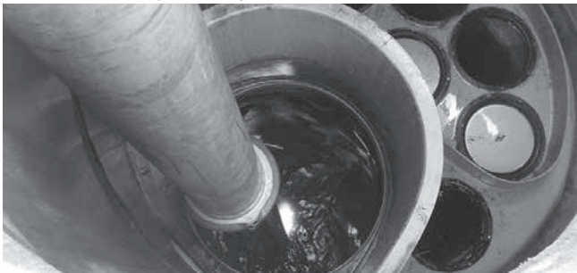
Vacuuming Sump Through MAW
