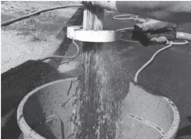
Vacuuming Sump Through MAW
