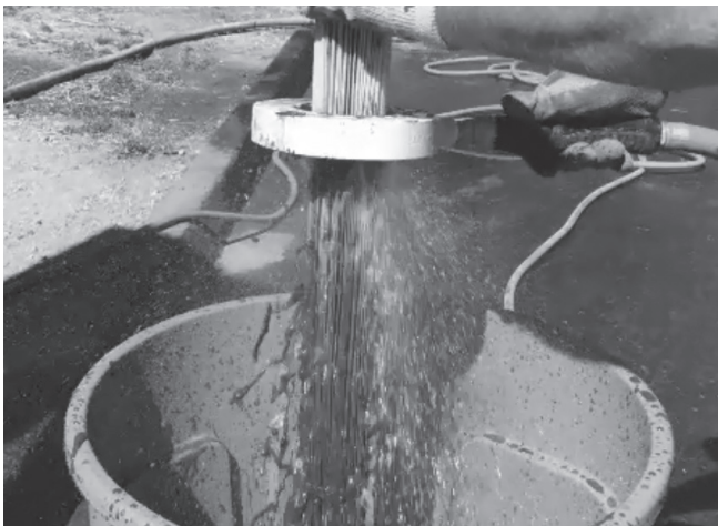
Vacuuming Sump Through MAW
