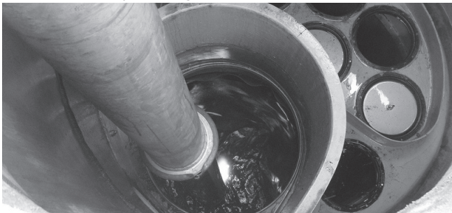
Vacuuming Sump Through MAW
