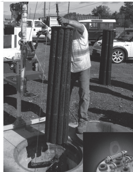
Cartridge Removal & Lifting Device
