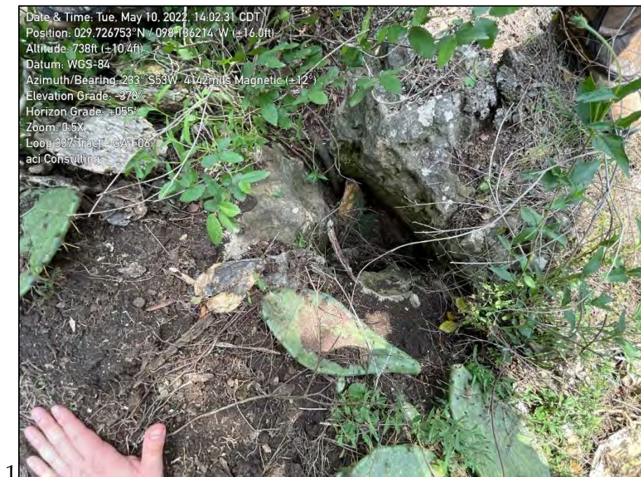
F06 before excavations.
