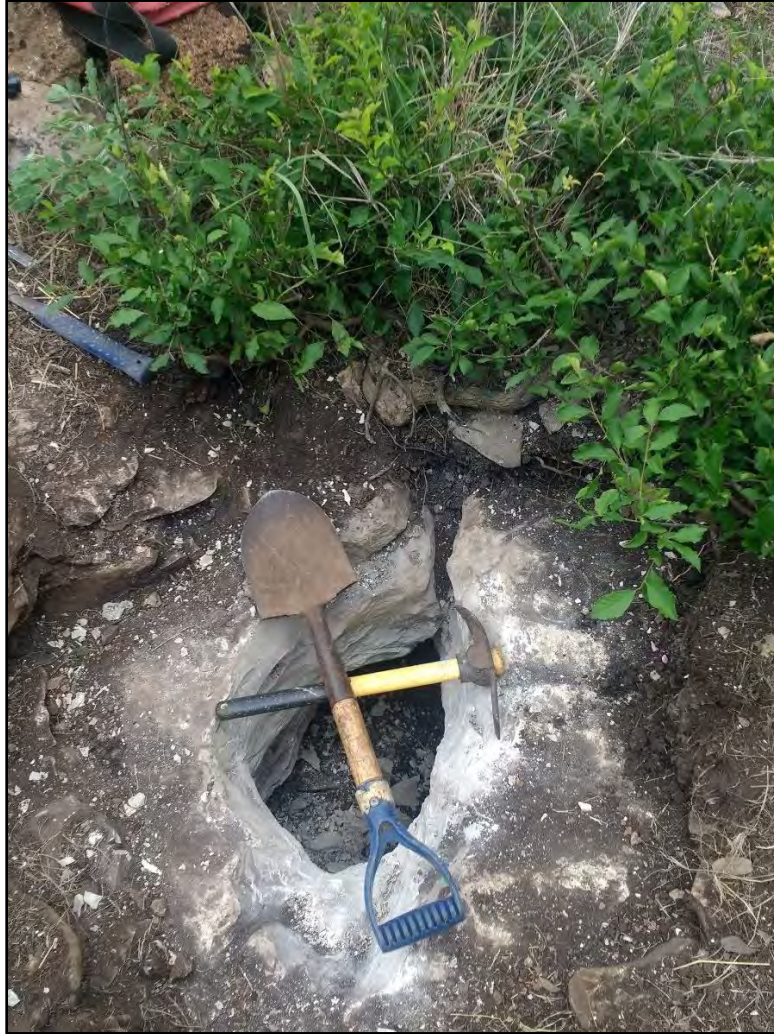
F21 after excavations.
