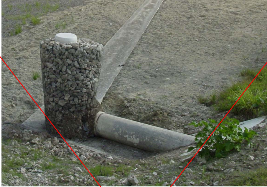
Figure 4 Detail of Trash Rack
