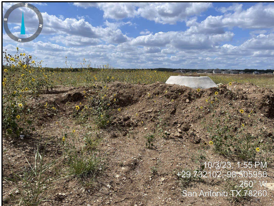
Photograph 4. Existing sewer line S-1.
