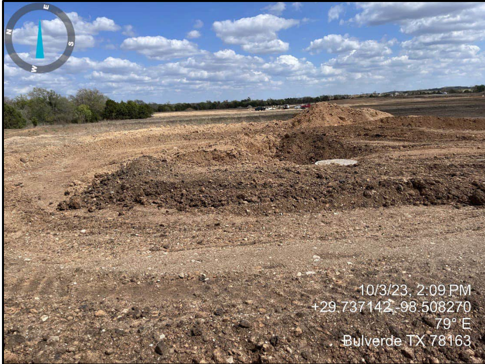
Photograph 3. Existing sewer line S-2.
