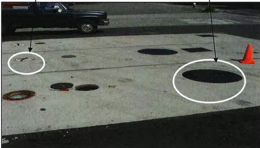
View of sump lids
