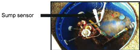
Sump sensor in contained turbine sump
