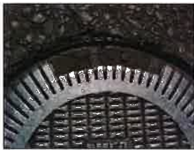
Cracked spill bucket lid
