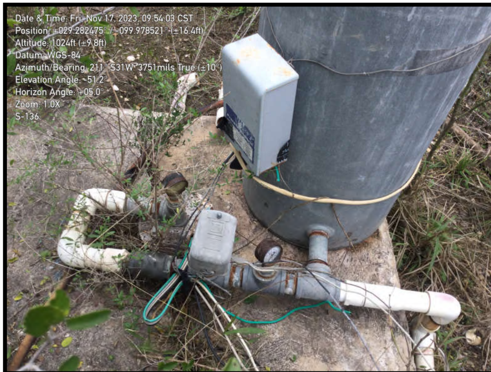
S-136: Manmade feature in bedrock, water well
