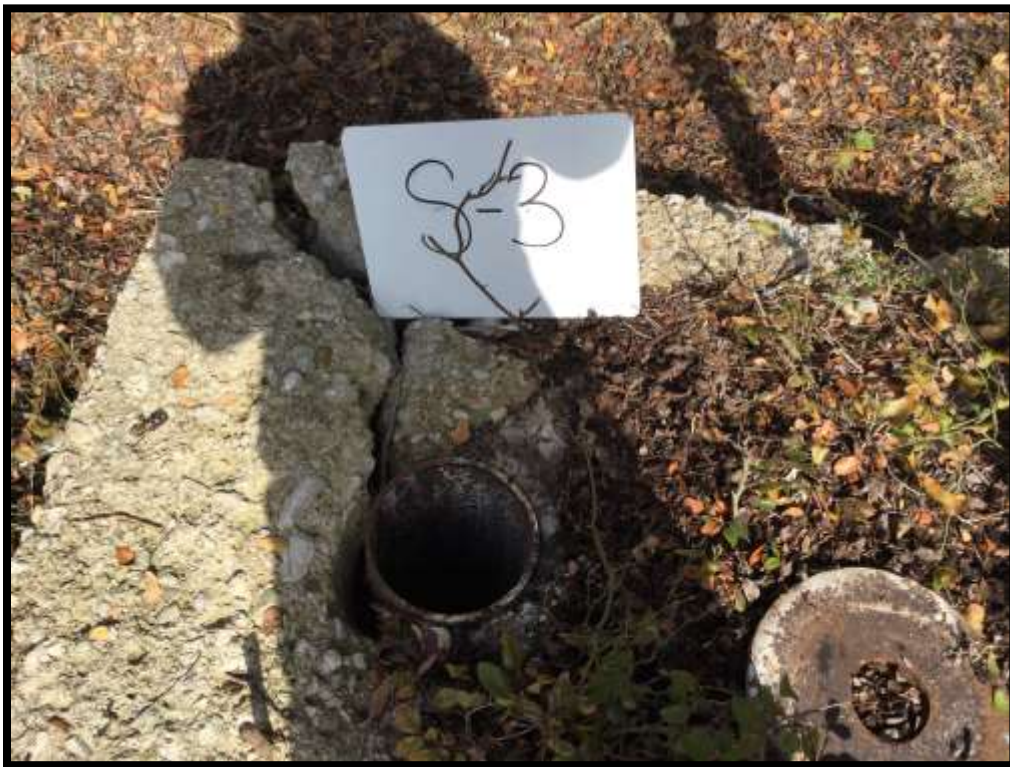
S-3: Uncapped well that is no longer in use.
