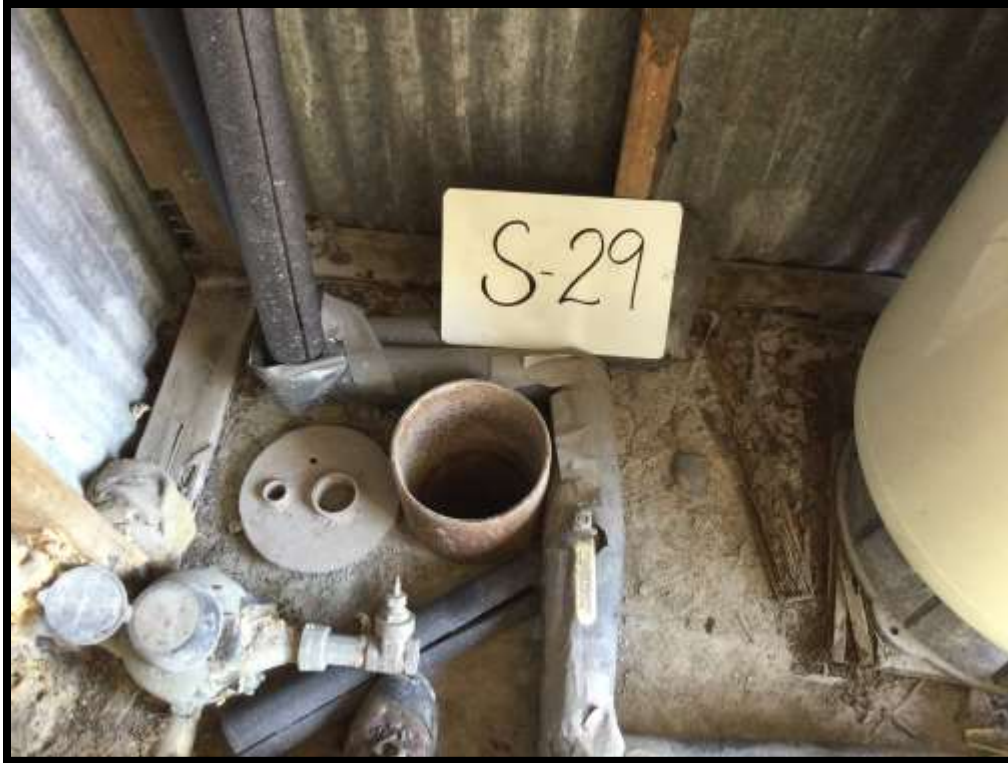
S-29: Water well (Tracking #87171) found uncapped inside a well house.
