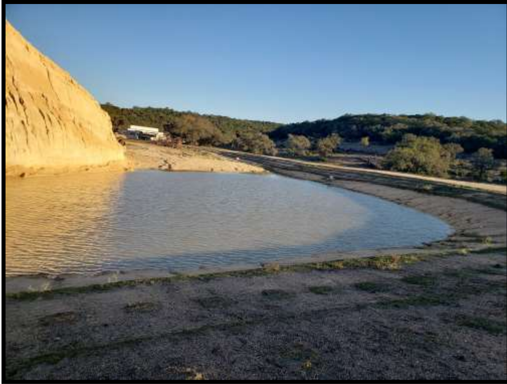
S-47: Stormwater pond classified as a non-karst closed depression.
