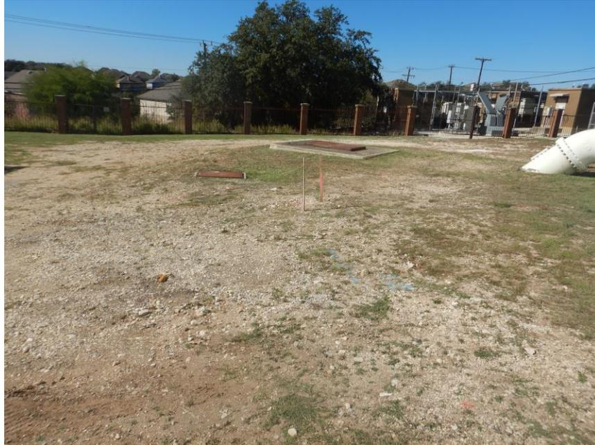
Photo 5. View facing west showing the likely surface connection from the existing underground 30-inch waterline that runs north to south within the project site. This photo also shows the location of the proposed 1 MG standpipe and additional underground pipe infrastructure.
