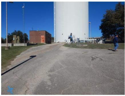
Photo 4. View facing north showing the existing 6 MG standpipe and associated pump/pipe infrastructure.
