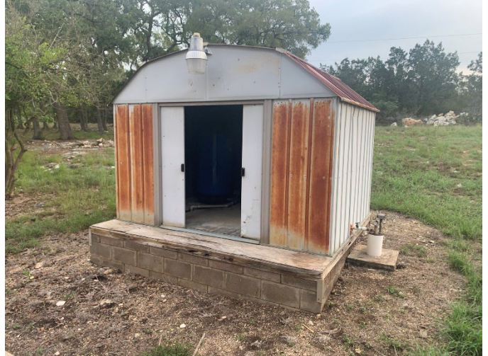
MB-4 Water Well In Front of Residential House
