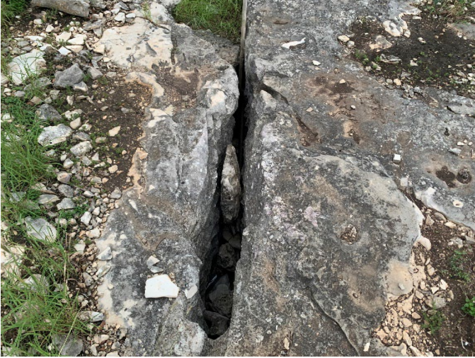
SF-1 Solution Enlarged Fracture
