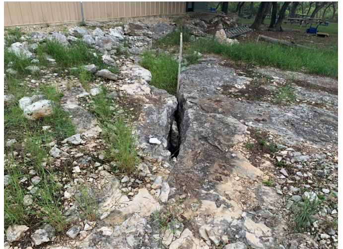
SF-1 Solution Enlarged Fracture Behind Commercial Fitness Building
