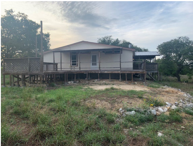
MB-5 Septic System Behind Residential House
