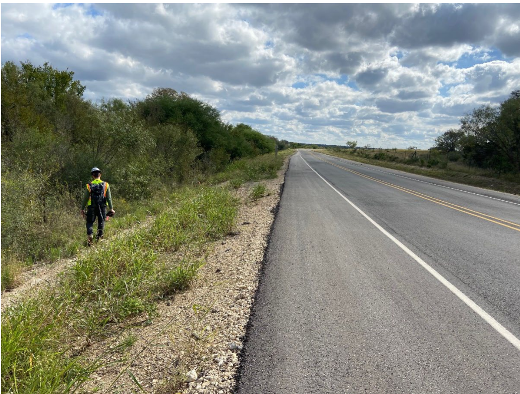
Photo 4. Roadway is not curbed or guttered, and water is conveyed via grassy swales or sheetflow off the project area. Facing south.
