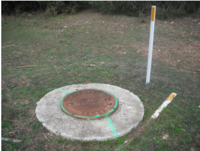
View of PRF # S-1014 near Area 1.
