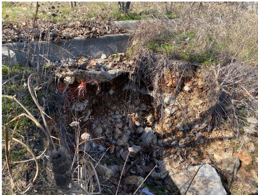
Photograph 10: Southwest facing view of the non-natural topographic depression originating from denudational processes exacerbated by the concrete stormwater drainage (MB-4), feature CD-1.
