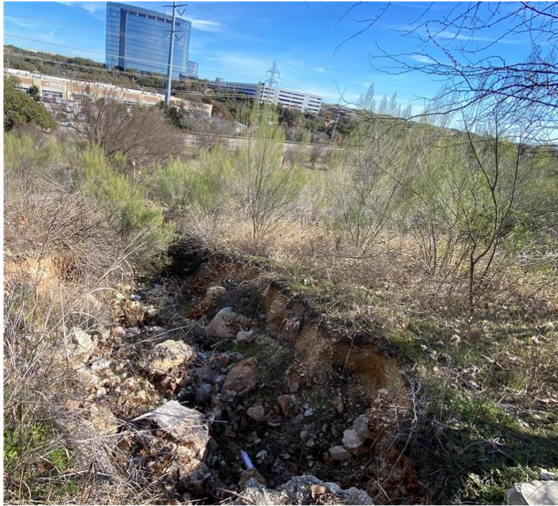
Photograph 9: Northeast facing view of the non-natural topographic depression originating from denudational processes exacerbated by the concrete stormwater drainage (MB-4), feature CD-1.
