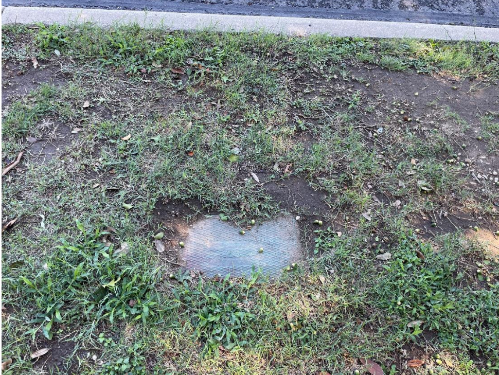
Photo #9: Typical view of electrical manway box (S-2) observed throughout the site.
