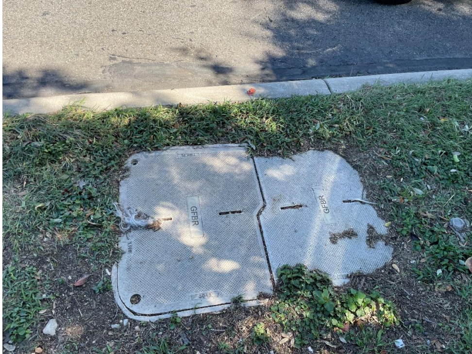
Photo #8: Typical view of GFR manway (feature S-1) observed throughout the site.
