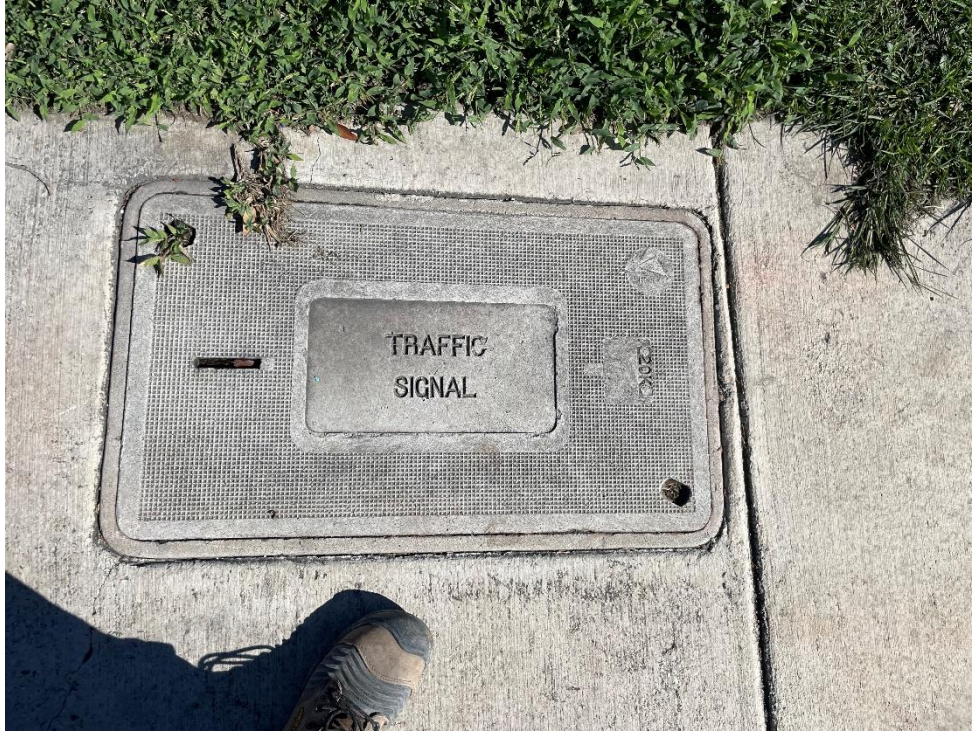
Photo #11: Typical view of a traffic signal manway (feature S-5) observed throughout the site.
