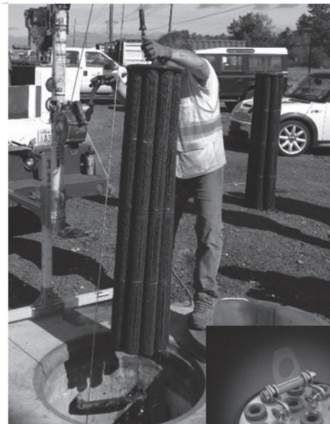
Cartridge Removal & Lifting Device
