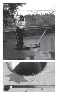
Inspection Utilizing Sediment Probe
