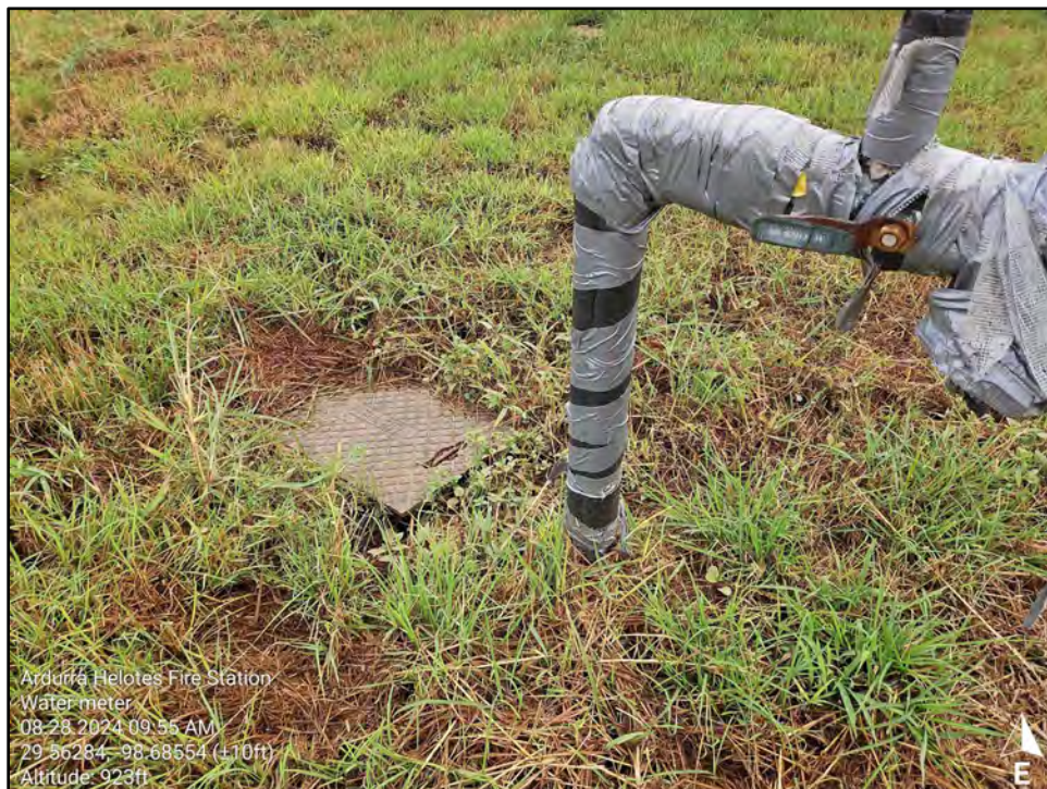
Figure 10. A water meter box and shut-off valve, an example of water line infrastructure, is visible in the northeastern part of the Survey Area near Bandera Road (MB-03).
