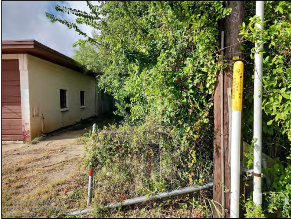
Figure 8. A natural gas line marker indicating the presence of a buried gas main, an example of natural gas infrastructure, is visible in the northwestern part of the Survey Area near Bandera Road (MB-02).
