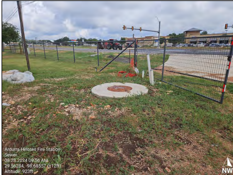
Figure 5. A manhole providing access to a City of Helotes sewer main, an example of wastewater sewer infrastructure, is visible in the northeastern part of the Survey Area near Bandera Road (MB-01).
