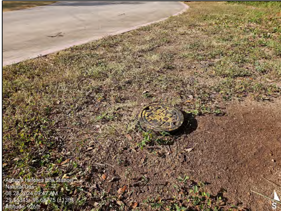
Figure 6. A cover providing access to an underground natural gas line, an example of natural gas infrastructure, is visible in the northwestern part of the Survey Area near the access road to Helotes Fire Station (MB-02).
