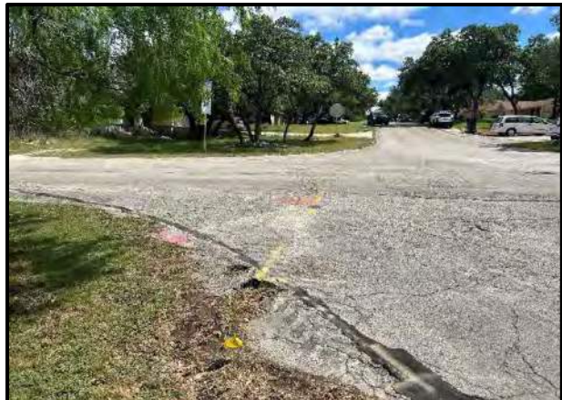
Gas line paint markings (i.e., yellow). View to the northwest from Pipestone Drive.
