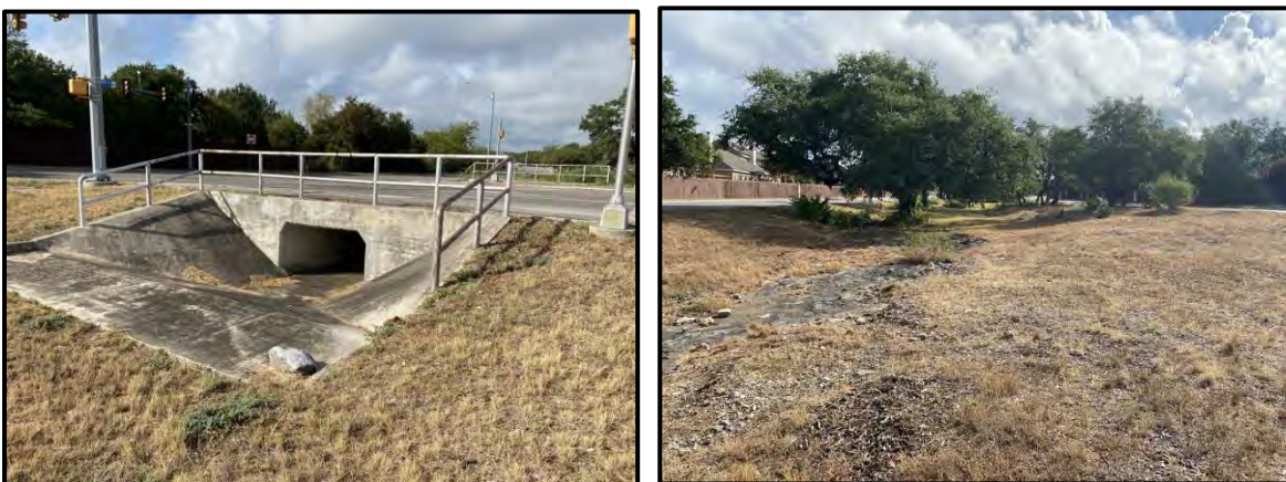
Left image: Box culvert where Roan Park crosses the median of Evans Road near the southwest end of the Project (view to the east). Right image: general view of the Evans Road median on the southwest portion of the Project where erosion has exposed bedrock (view to the northeast).
