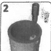
Lift float with cable to simulate fill
