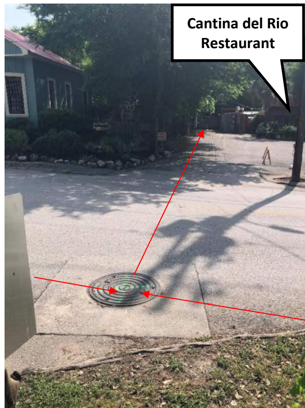
Figure 8: Manhole in Gruene Road with 12" Gravity Sanitary Sewer to Siphon Structure (View to SW)
