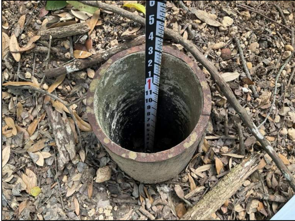
Photo 4. Feature 6. Unknown, unmapped pipes on a hillslope east adjacent to Gruene Road to the east of the Guadalupe River. The pipe was filled with soil and organic debris and could only be probed to a depth of 1.25 feet.
