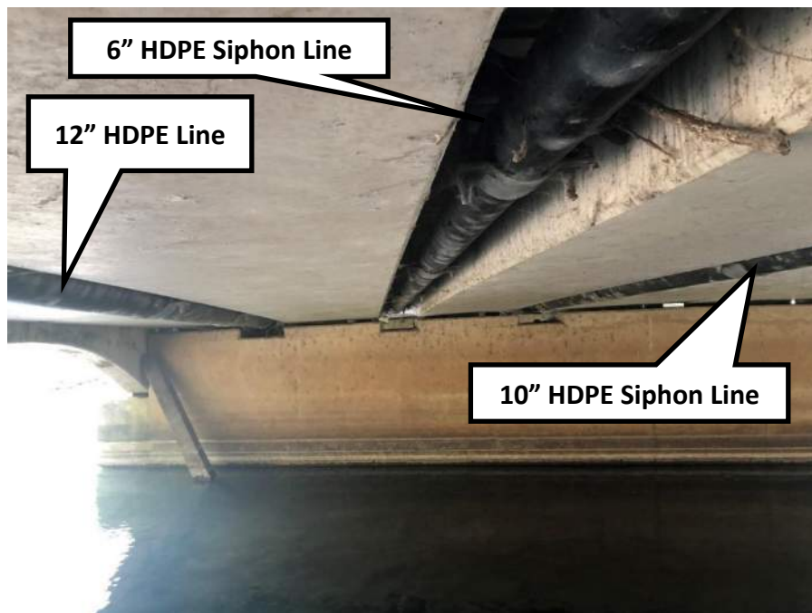
Figure 15: Siphon Lines Underneath the Gruene Road Bridge (View to SW)
