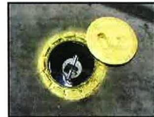
Circular spill bucket lid pulled back to show the fill port with a spill bucket
