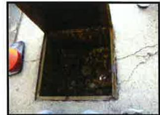
Square steel sump lid pulled up to show the inside of an uncontained turbine sump
