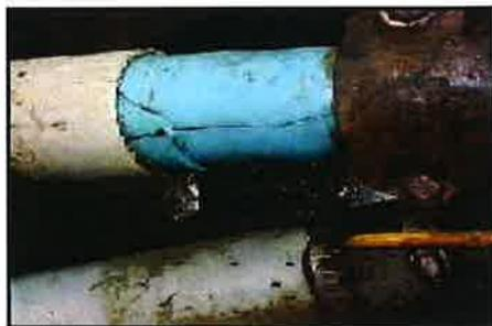
Flexible piping is cracked
