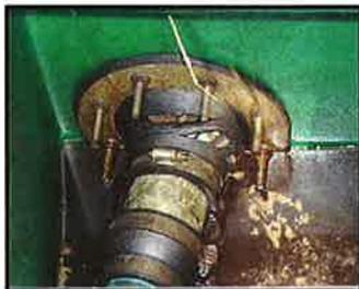
Sump penetration seals in poor condition
