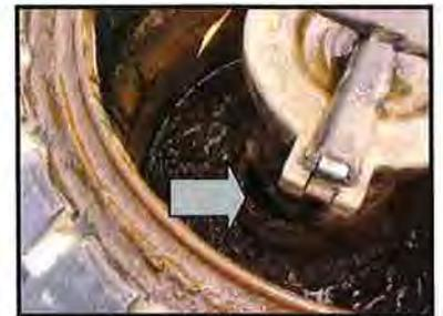
Spill bucket in poor condition – note the gap between the spill bucket and the fill pipe
