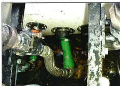
Metal flexible connector is twisted due to growth of flexible plastic piping
