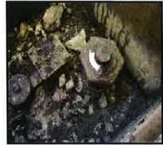
Equipment and metal piping covered with dirt in uncontained sump
