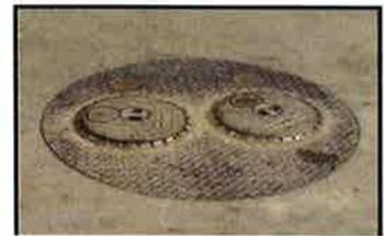
Fill and vapor recovery lids installed within a larger sump lid
