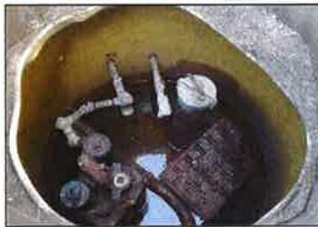
Contained sump with liquid and debris
