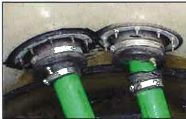
Test boots positioned at sump wall, right test boot is torn
