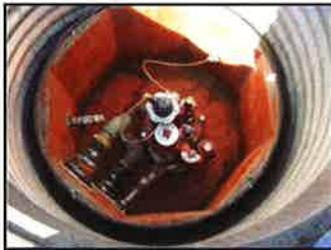
Dry, debris-free contained turbine sump
