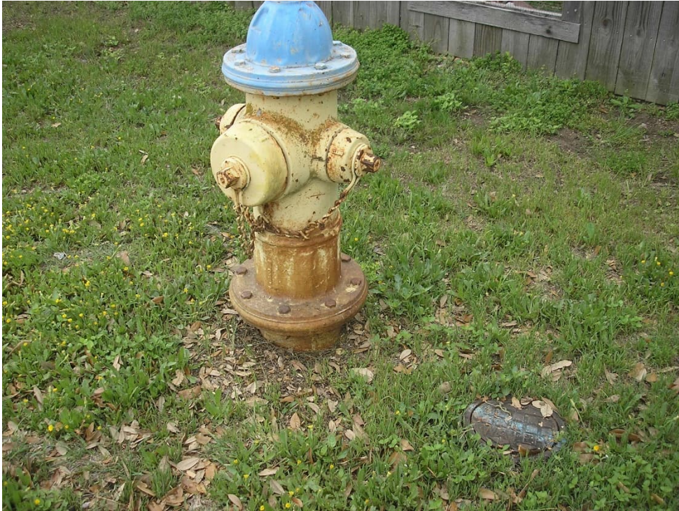
Photo #5: View of fire hydrant and 6-inch marked valve cover associated with feature S-2 in the vicinity of the eastern-central portion of site east of the intersection of Stonepath Drive.
