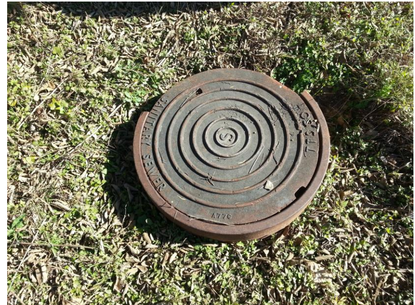
Photo #4 Typical view of one of the few sanitary sewer manhole covers (feature S-6) noted throughout the site.
