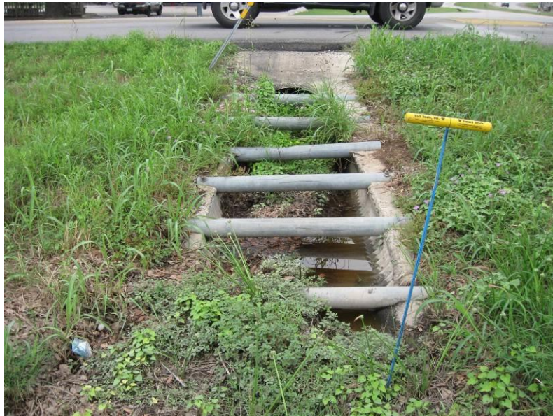
Photo #3 View of non-karst closed depression (drainage culvert, feature S-8).
