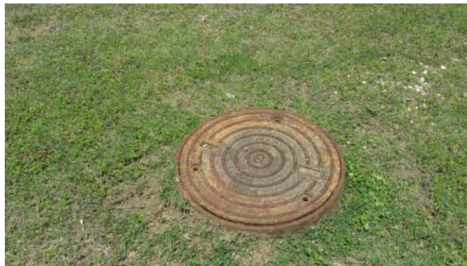
View of a Sanitary Sewer Manhole Cover, Potential Recharge Feature # S-6.
