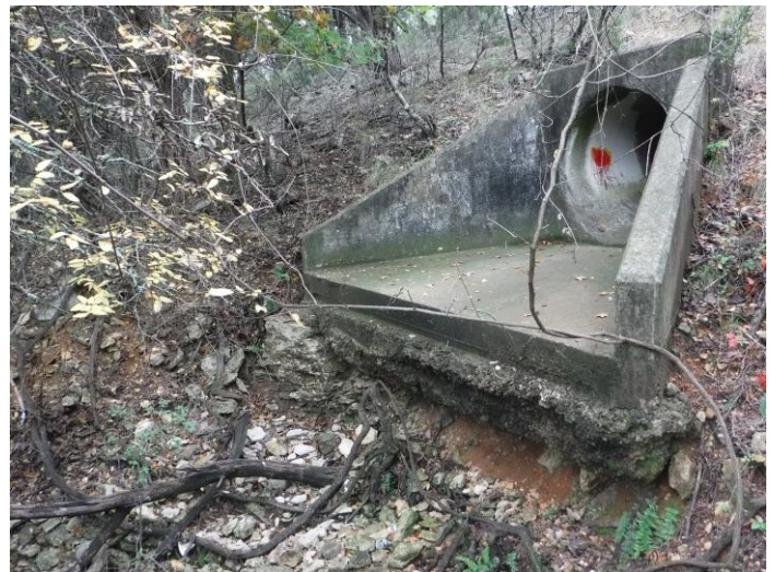
Photo #8 – View of the land surrounding F-4, including a concrete storm drain.
