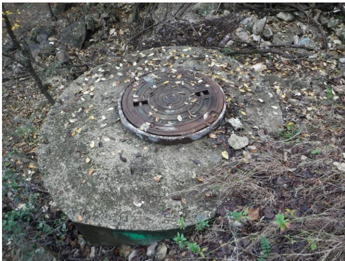
Photo #7 – View of Feature F-4, a SAWS sanitary sewer manhole cover.
