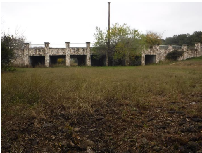
Photo #19 – View of the land surrounding S-2, including a storm drain beneath Gold Canyon Drive.
