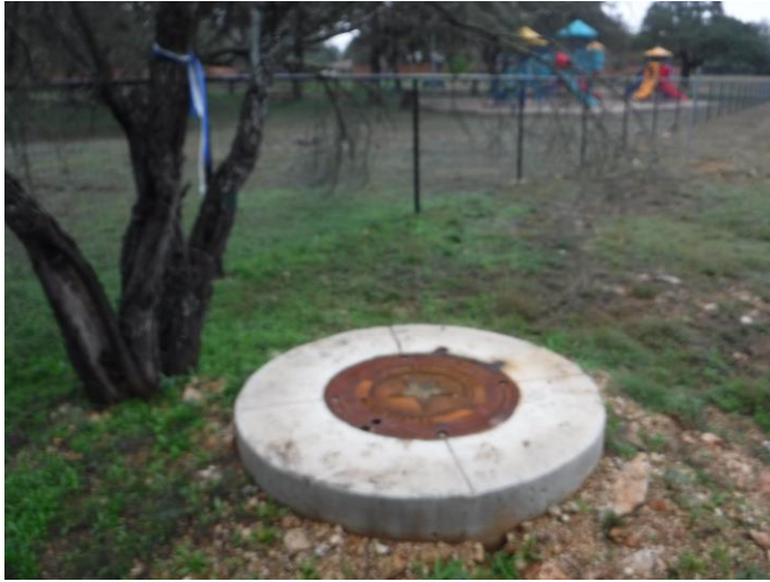
Photo #1 – View of Feature F-1, a SAWS sanitary sewer manhole cover.
