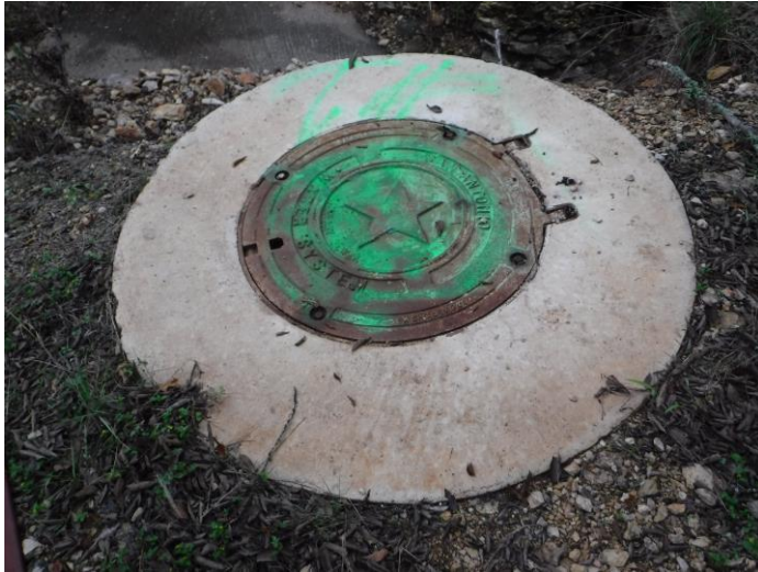
Photo #5 – View of Feature F-3, a SAWS sanitary sewer manhole cover.
