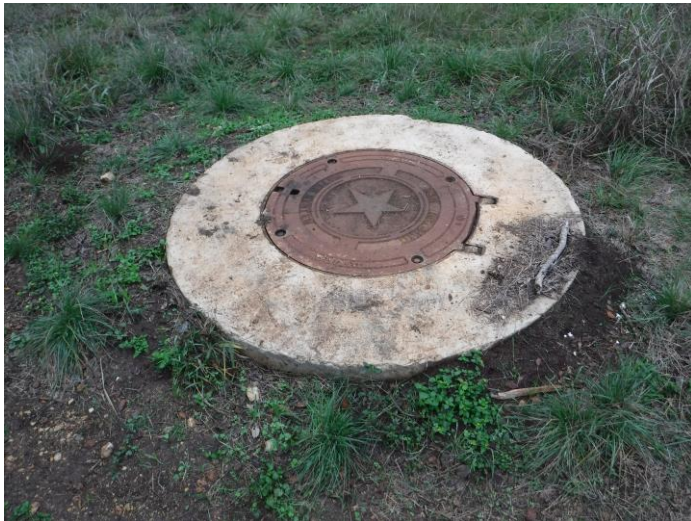
Photo #3 – View of Feature F-2, a SAWS sanitary sewer manhole cover.
