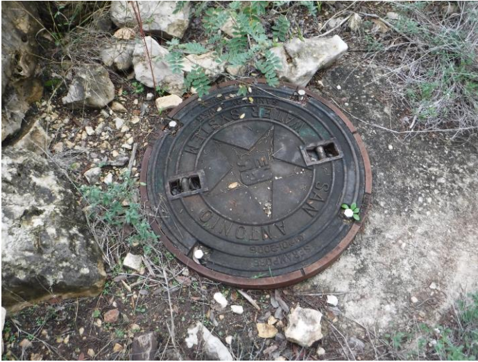
Photo #9 – View of Feature F-5, a SAWS sanitary sewer manhole cover.
