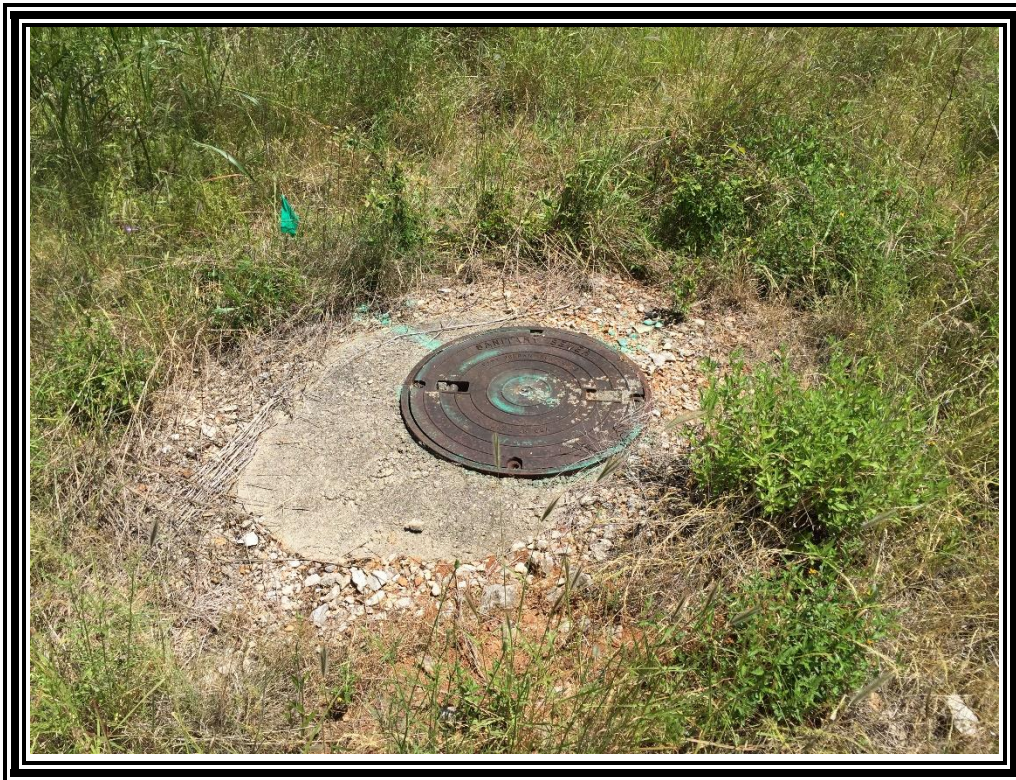
5. View of manhole feature S-1 on the northern portion of the site (29-43-20; 98-10-37.9).
