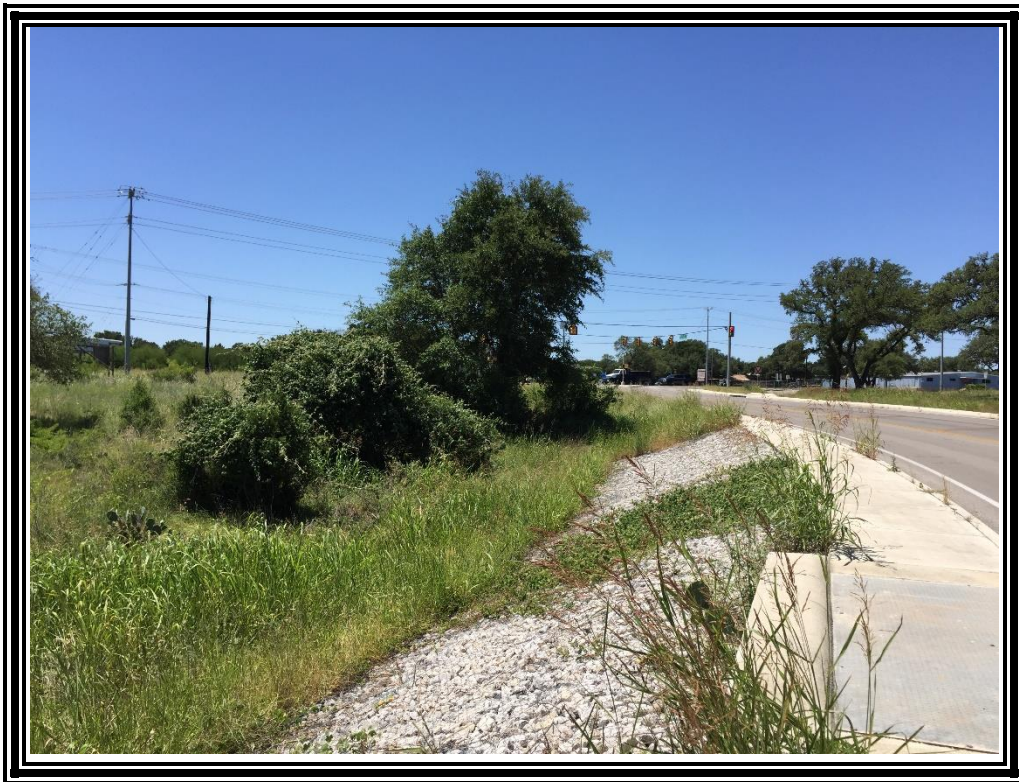
8. View southwest along Alyssa Way from the northwest corner of the site.
