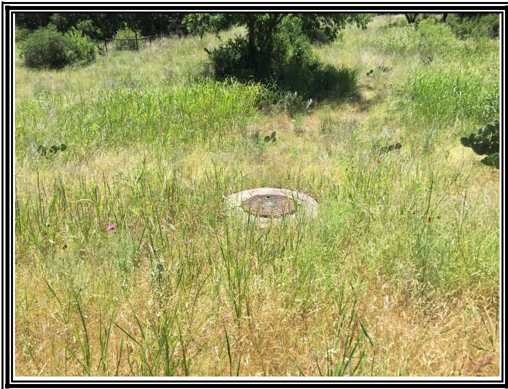
10. View of manhole feature S-2 located at 29-43-20; 98-20-34.8, near the northwest corner.
