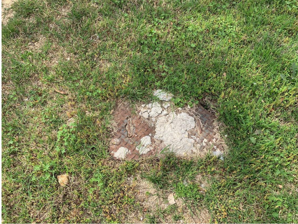
Photo #13: View of water meter box at the location of feature S-7.
