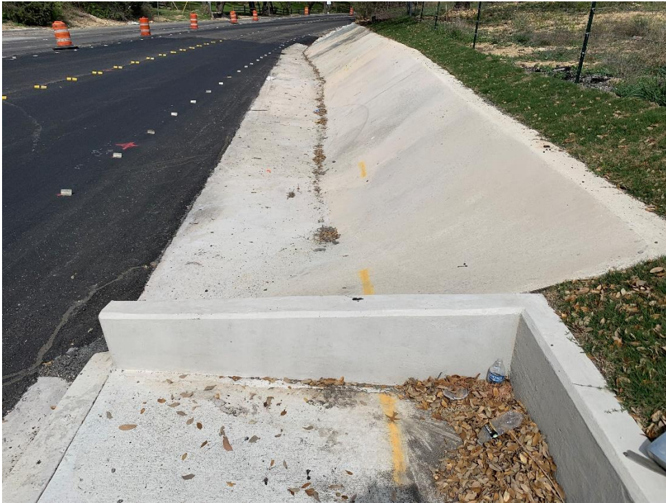
Photo #11: View of marked gas line (yellow paint marks) at the location of feature S-6.
