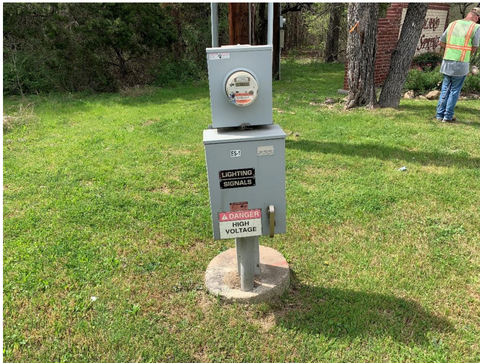
Photo #18: View of electrical meter box and marked electric line at the location of feature S-12.
