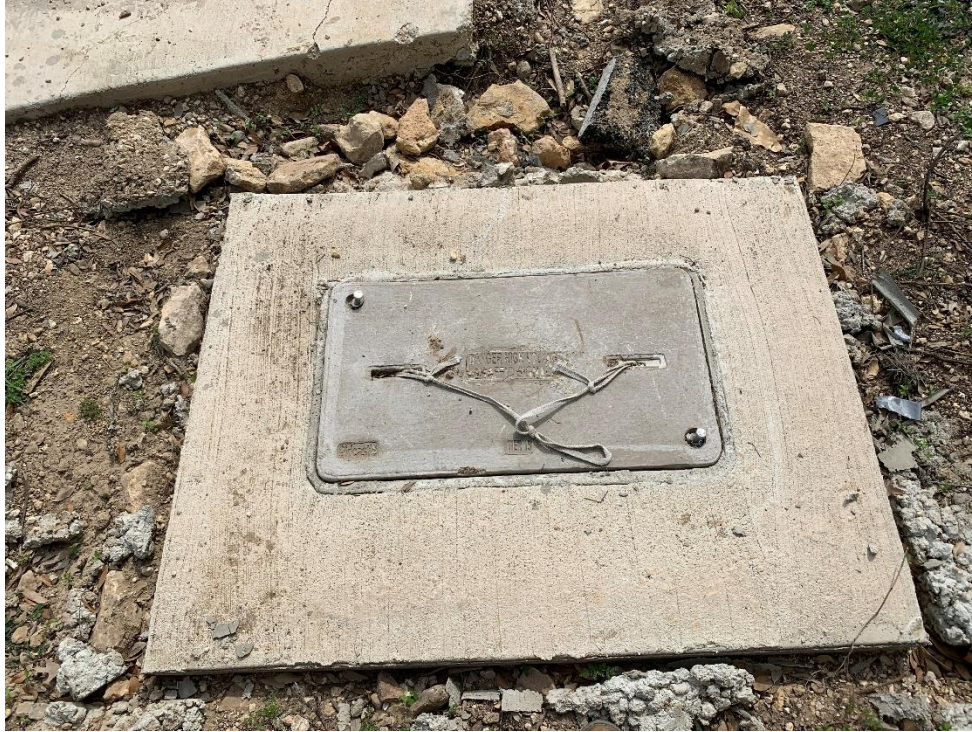
Photo #15: View of communication manway box at the location of feature S-8.
