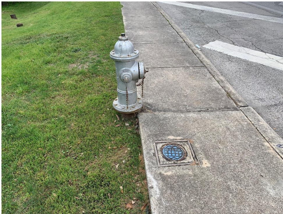
Photo #14: View of marked water manway and fire hydrant at the location of feature S-7.
