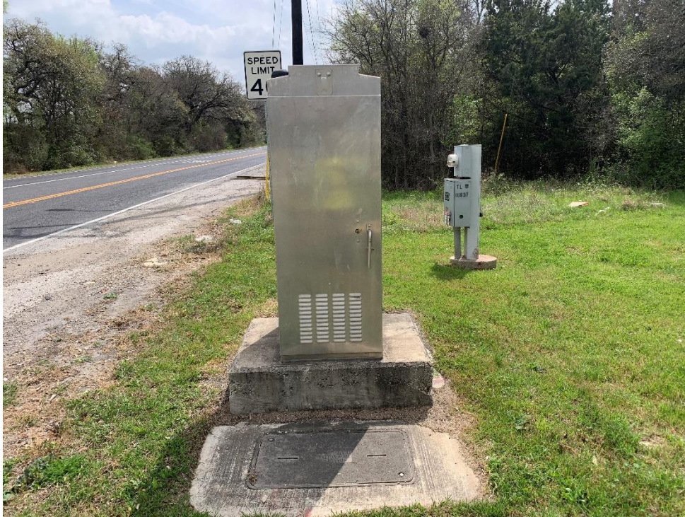
Photo #17: View of traffic signal utility boxes and marked electric line at the location of feature S-11.
