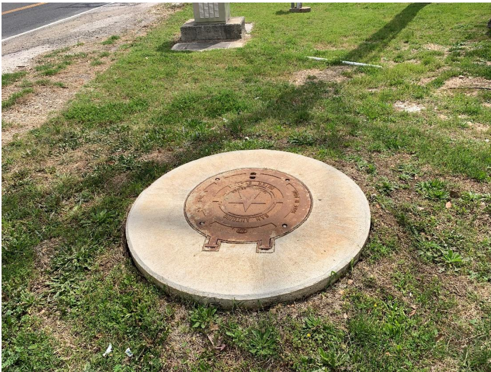
Photo #6: View of sewer manway at the location of feature S-3.
