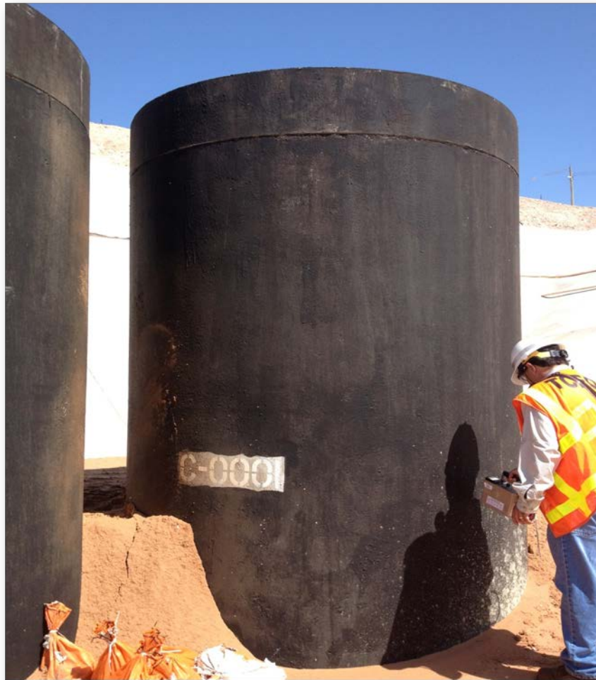
Figure 4-1. Cylindrical Modular Concrete Canister Used in the CWF (TCEQ, 2014).
