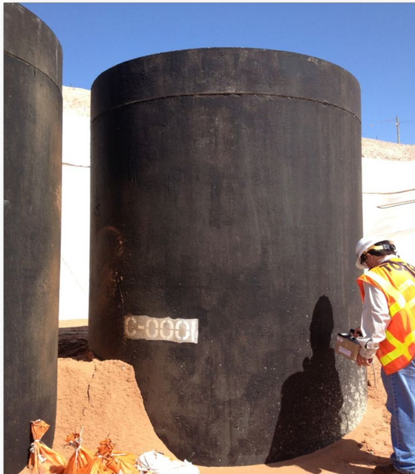
Figure 10. Cylindrical Modular Concrete Canister Used in the CWF (TCEQ, 2014)
