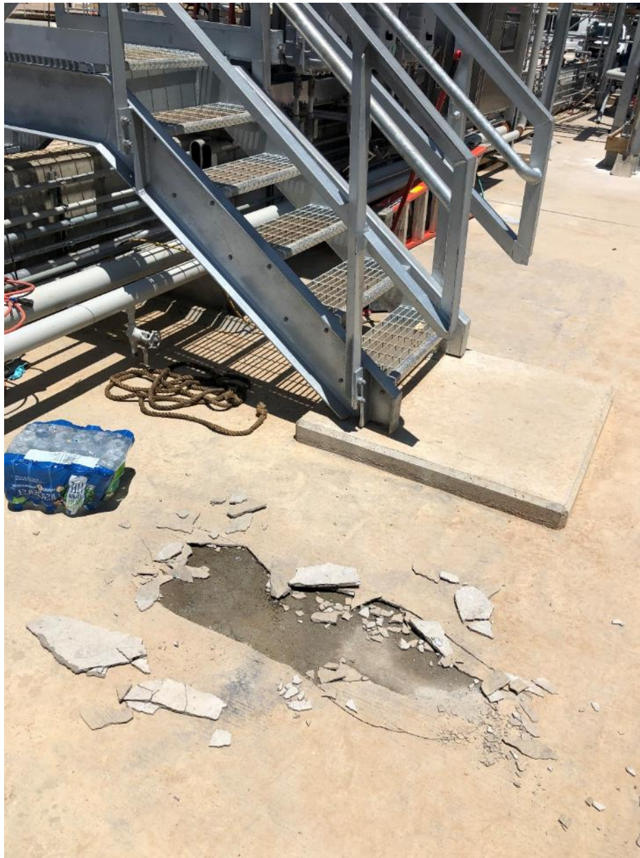
Location of superficial cracks in the northern portion of the secondary containment area. Facing north
