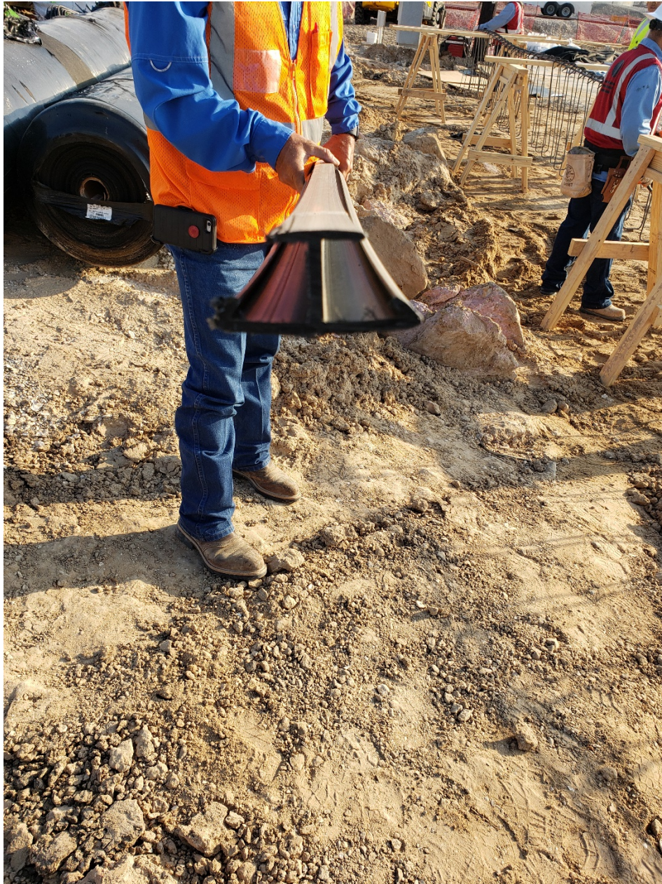
Geomembrane concrete anchoring support. Photograph taken facing southeast.
