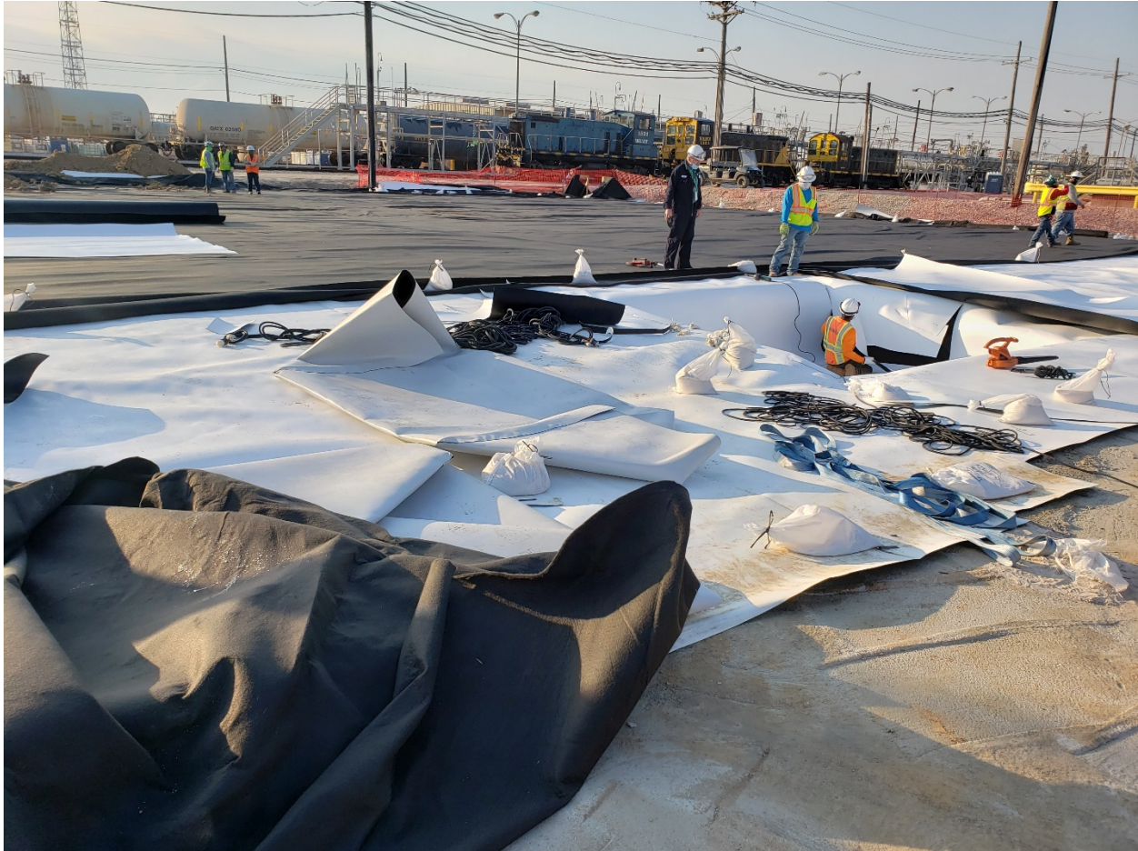
Geomembrane installation. Photograph Taken Facing South.
