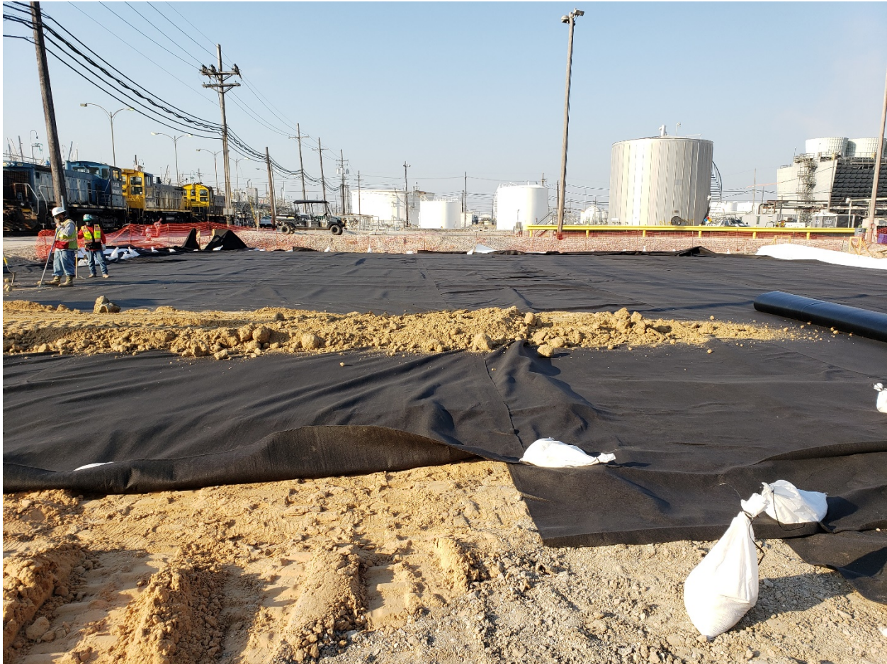
Northeastern side of the upper soil cover over geomembrane. Photograph taken facing southwest.
