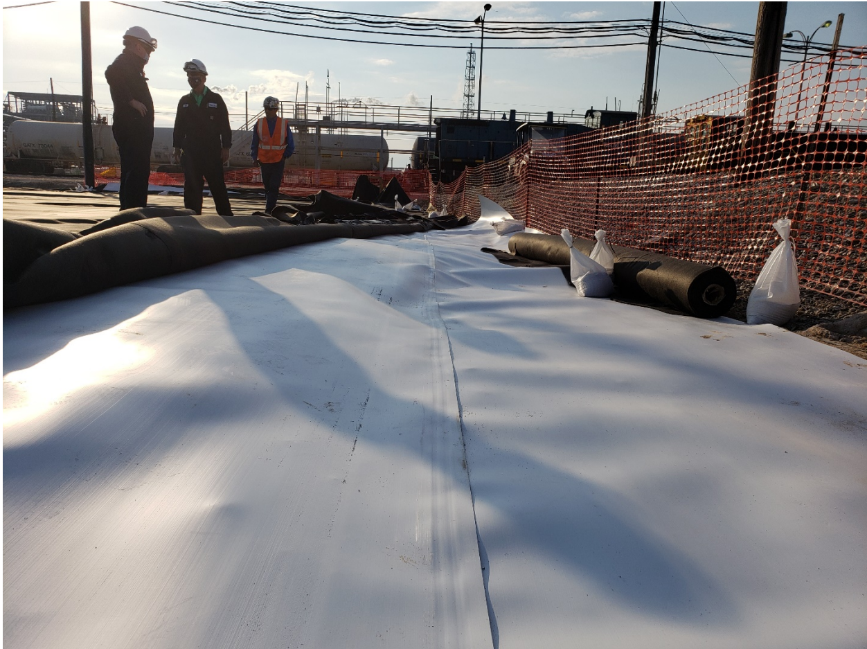
Eastern side of the geomembrane installation. Photograph taken facing southeast.
