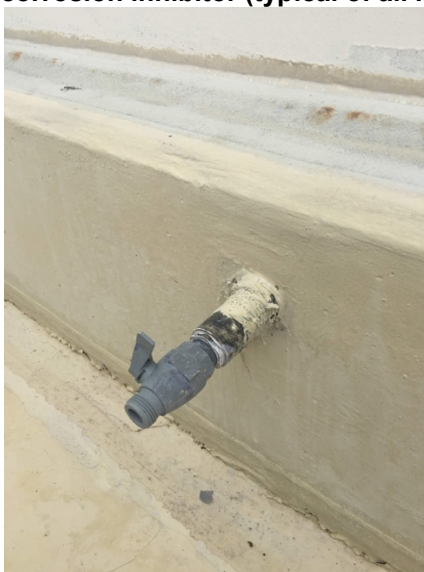
Electrical Resistance Probes on IWPf Tank 332T1-1.
