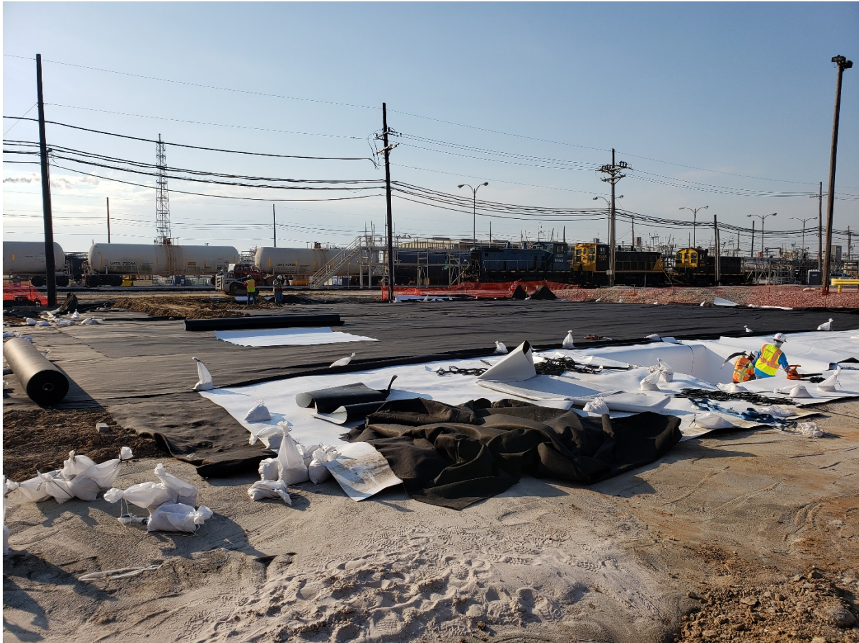
Geomembrane installation. Photograph Taken Facing South.
