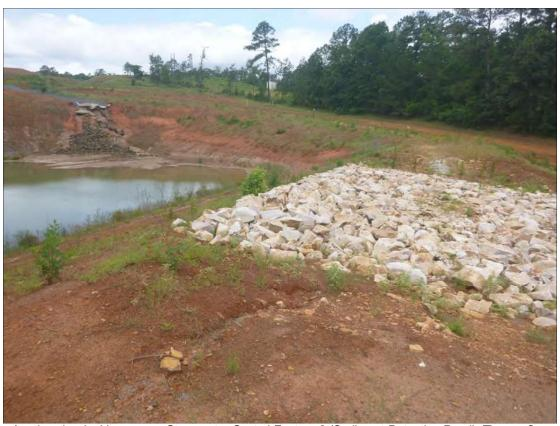
Another view looking across Stormwater Control Feature 2 (Sediment Detention Pond). The overflow spillway is visible on the right side of the photograph.
