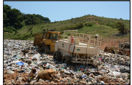
Proper orientation of equipment on slope
