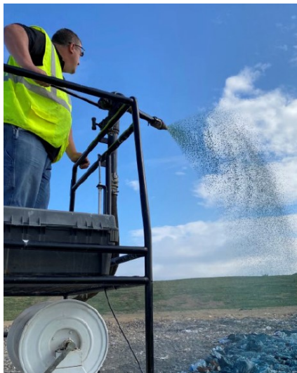
Application of VERDac Pellets via Deck -Mounted Discharge Wand
