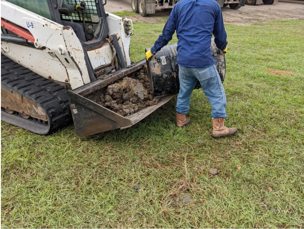
Cuttings Disposal and Transport to Transfer Station
