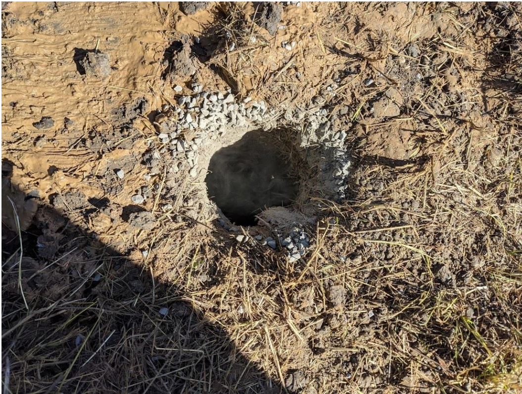
Backfilling Borehole With Granular Bentonite
