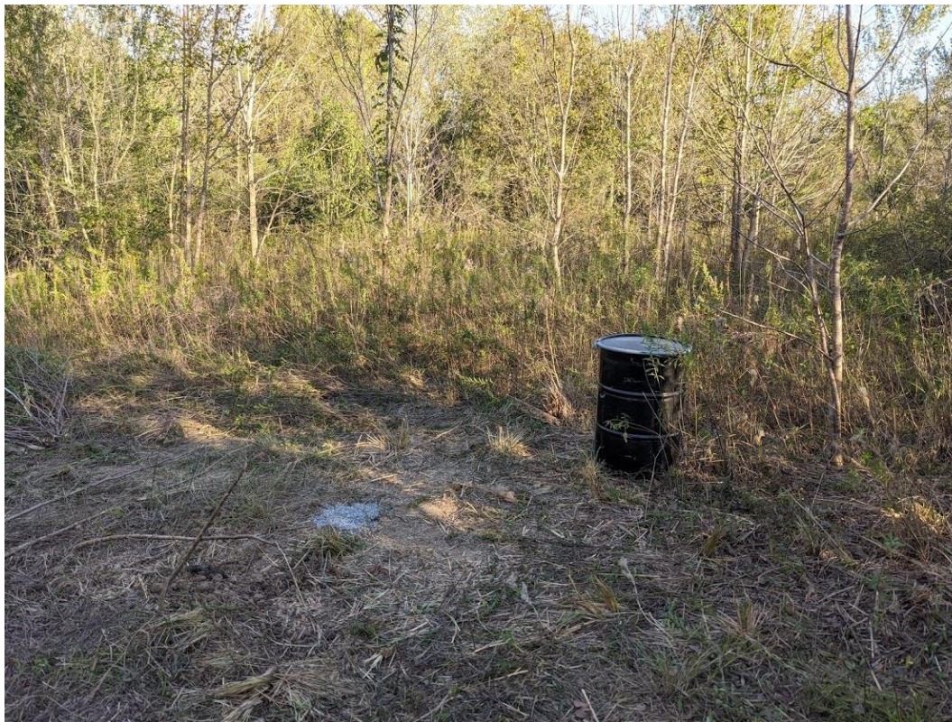
Bentonite Backfilled Borehole and Cuttings Drum
