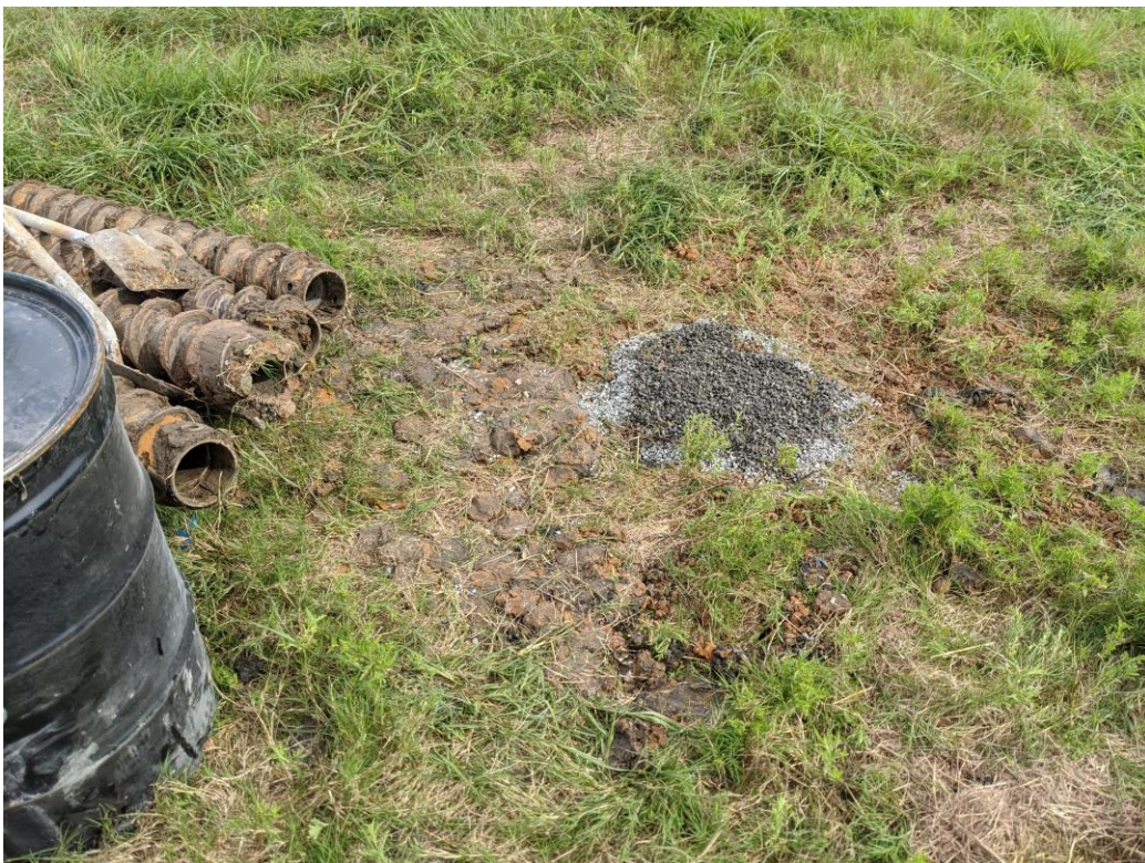
Bentonite Backfilled Borehole
