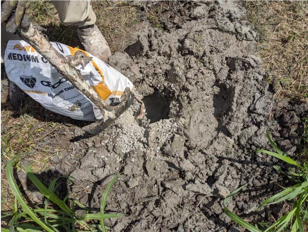
Backfilling Borehole with Granular Bentonite
