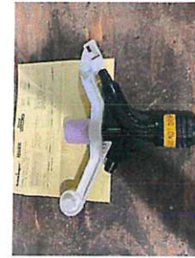
INSTALLED SPRINKLERS SENNINGER 8025HR-1 IMPACT SPRINKLER W/ #52 NOZZLE (1/2")
