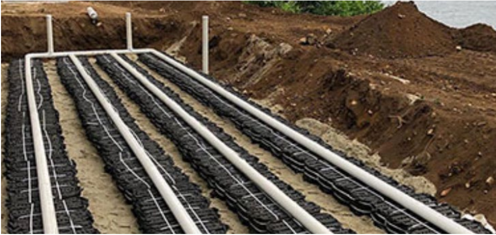
Figure 2 – Installation Configuration for Laterals and Chambers
