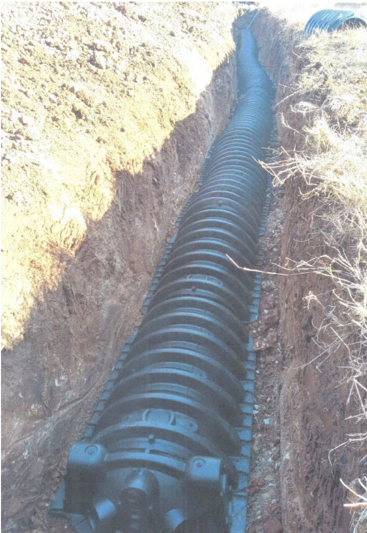
Figure 1 – Example of Interceptor Gravel-less Chamber
