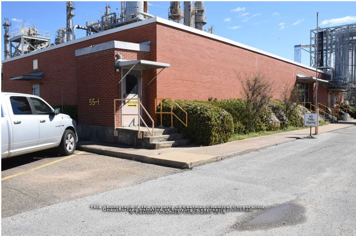
(52) Bld. No. 55 – Camera facing northeast
