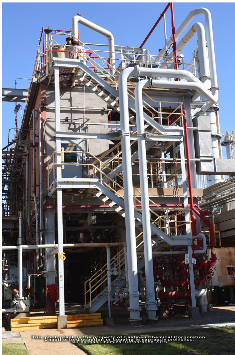
(18) Bld. No. 16 – Camera facing north
