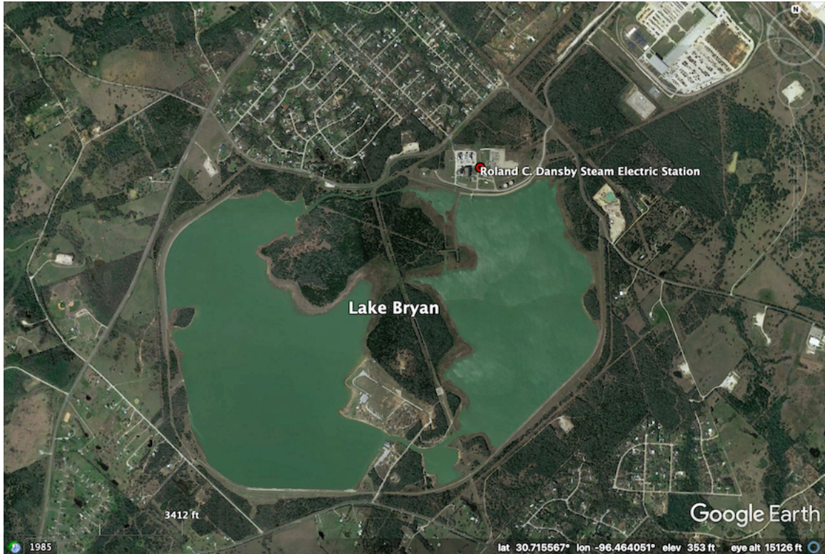
Facility Aerial Overview – Power Plant and Lake Bryan
