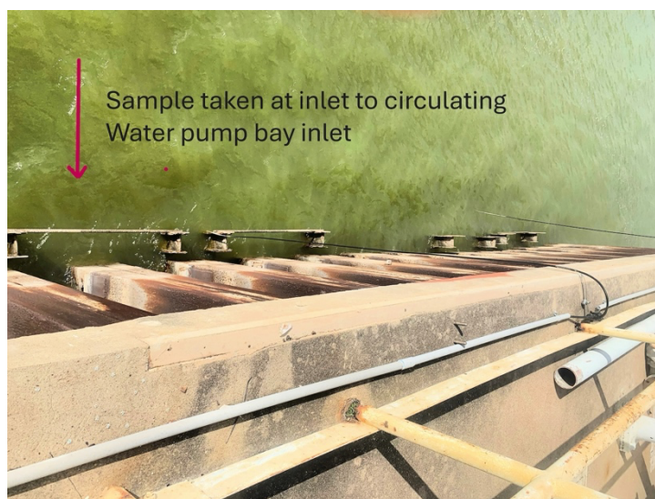
Photo 2. Intake Sample Point
