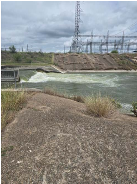
Photo 6: Outfall 301 (future) looking north
