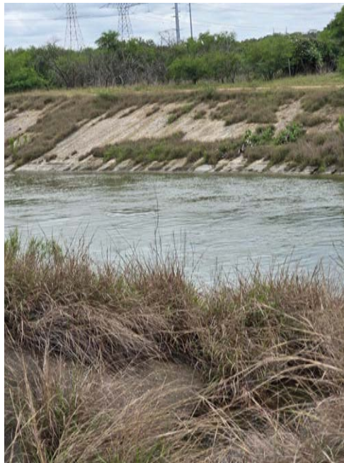
Photo 8: Outfall 401 (future) view across channel
