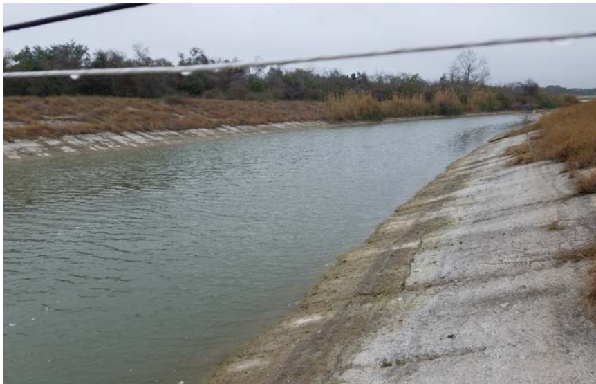
Photo 3: Downstream of Outfall 001
