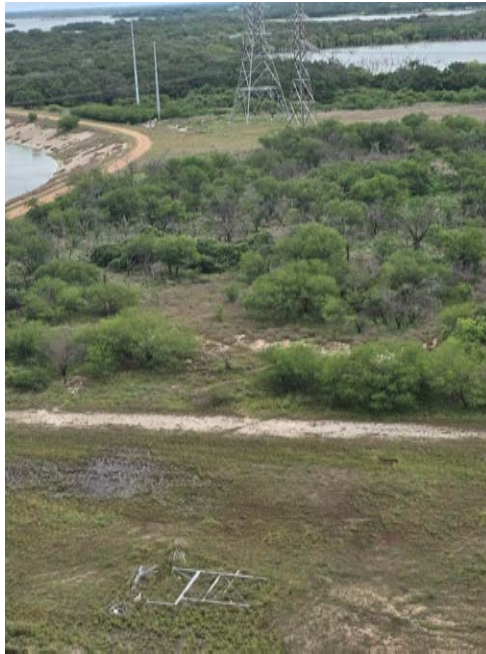
Photo 10: Site for new Retention Pond
