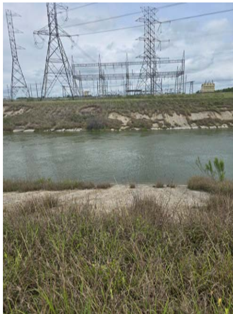
Photo 9: Outfall 401 (future) view from south
