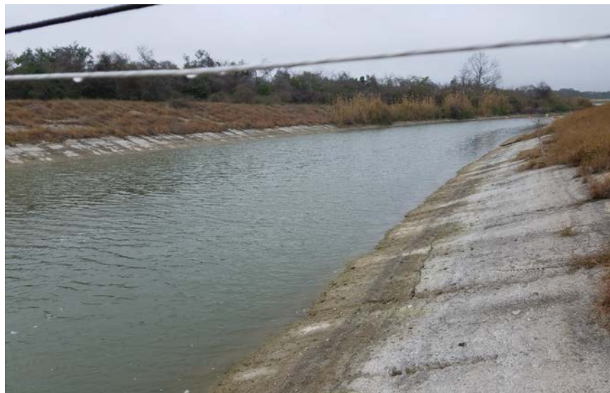
Photo 3: Downstream of Outfall 001
