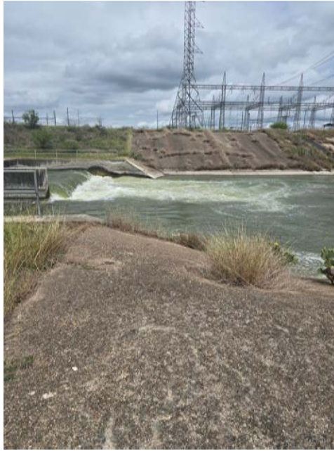
Photo 6: Outfall 301 (future) looking north
