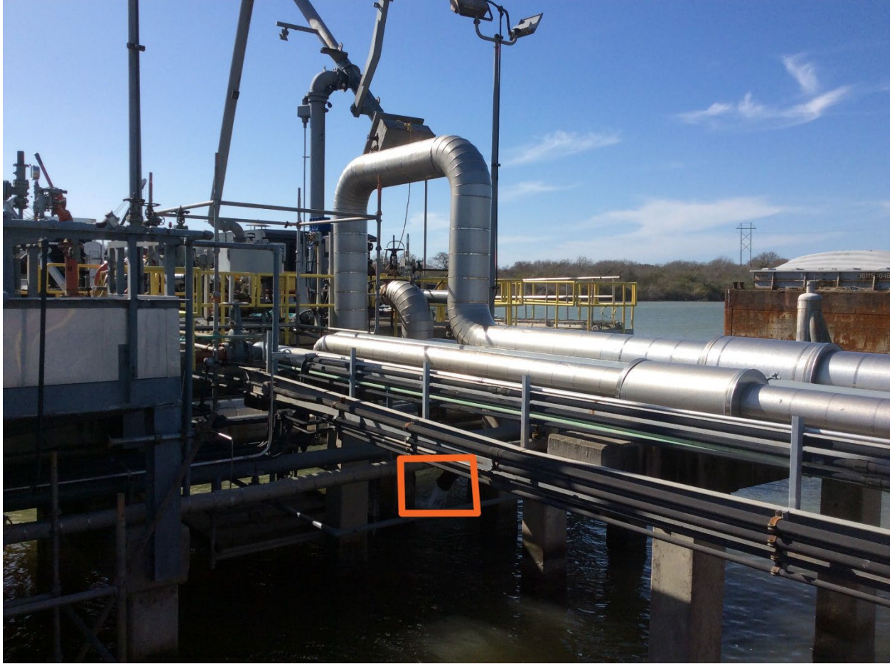
Fig 2. 001 Final discharge point facing northwest.
