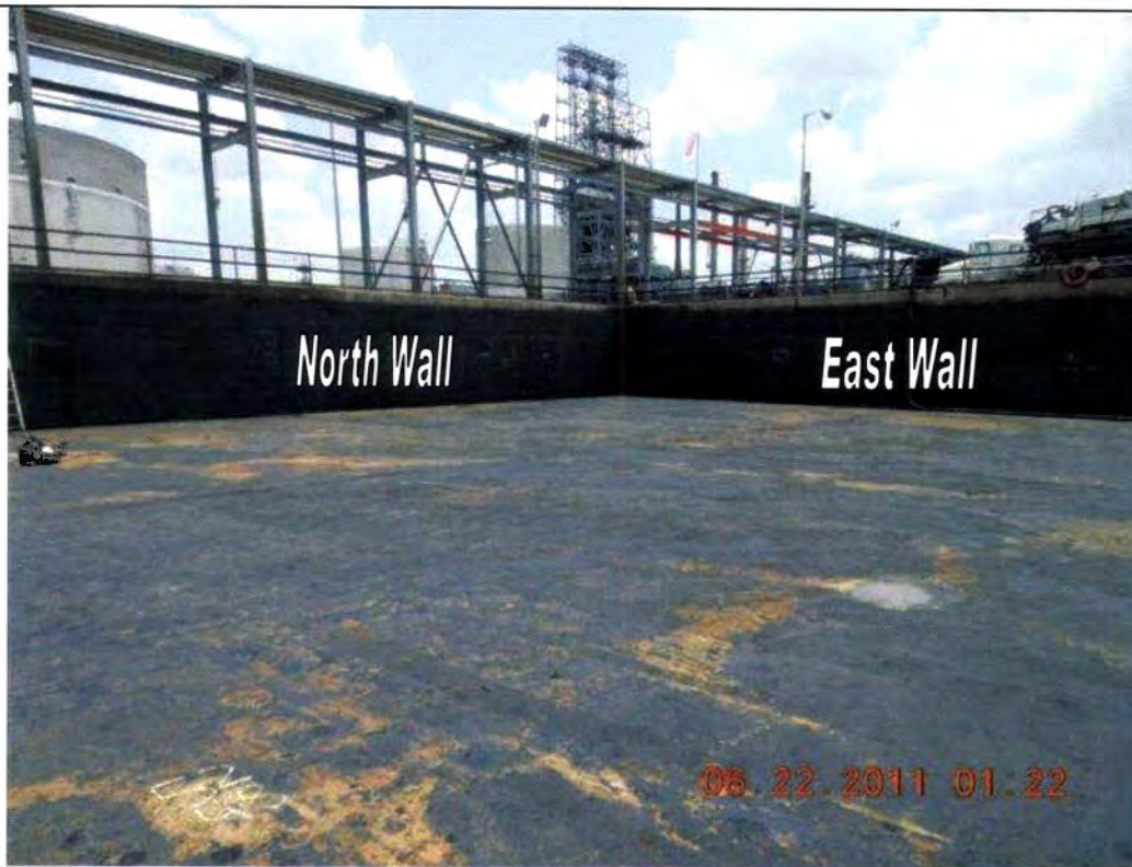
Photograph 12. Overview of the Northeast corner of the West Rain Basin.
