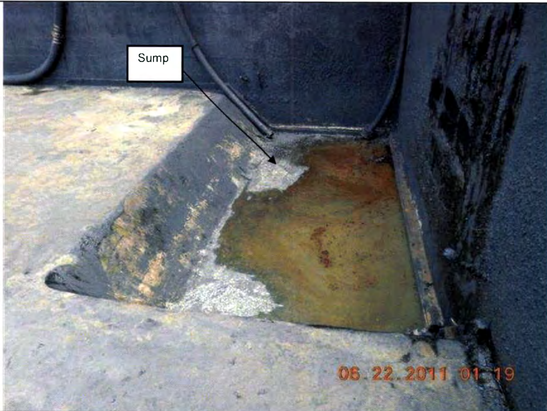
Photograph 7. View of Sump on the Southeast corner of the West Rain Basin.
