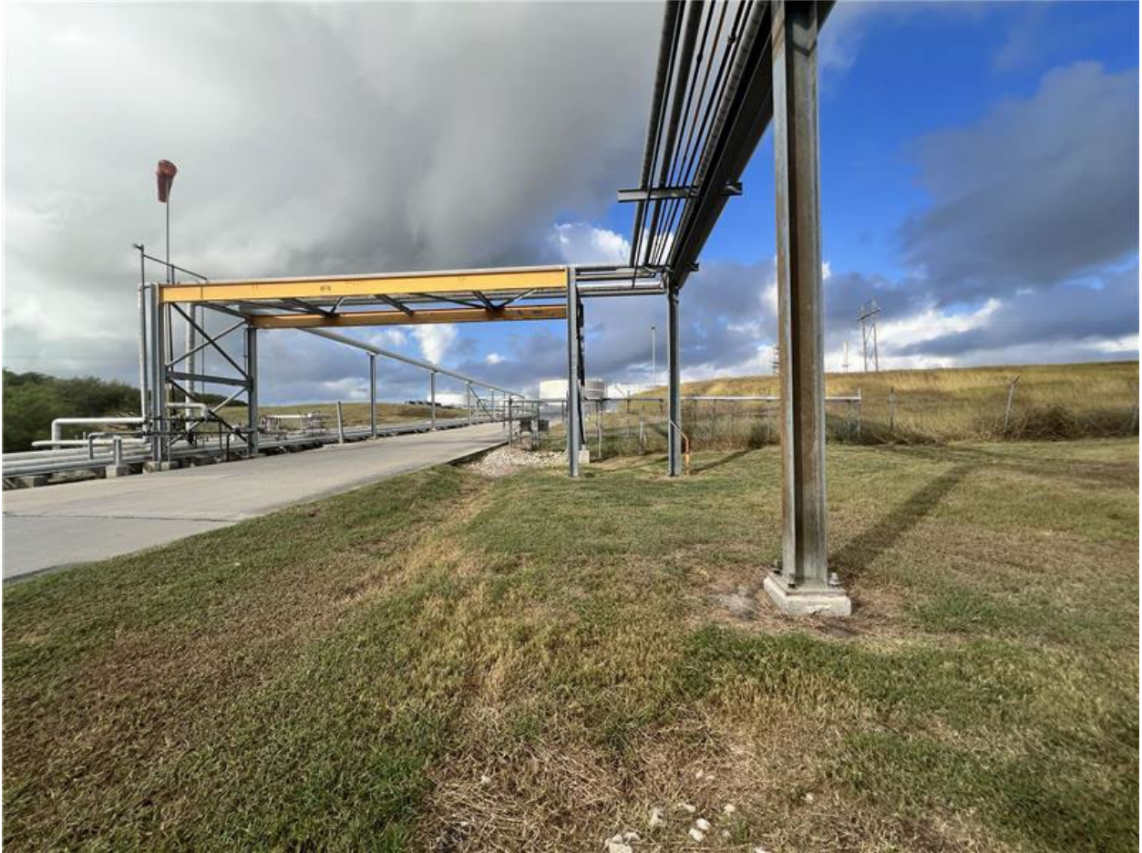
Fig 7. 003 final discharge point facing north.
