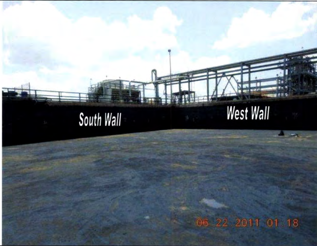
Photograph 3. Overview of the Southwest corner of the West Rain Basin.
