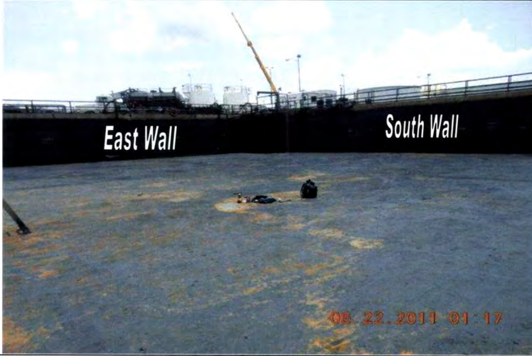
Photograph 1. Overview of the Southeast corner of the West Rain Basin.
