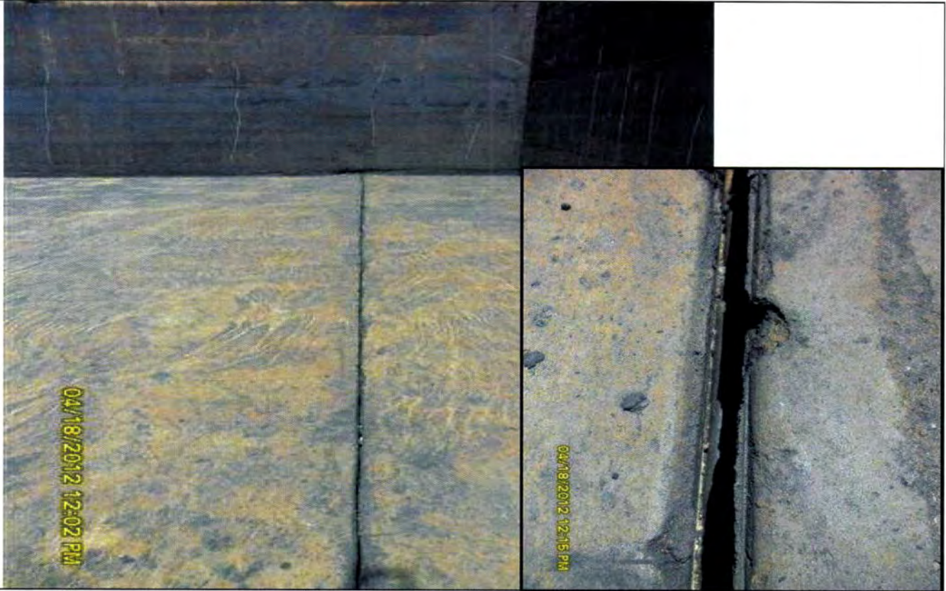
Photograph 11. View of East Expansion Joint within East Rain Water Basin Base Slab from South.
