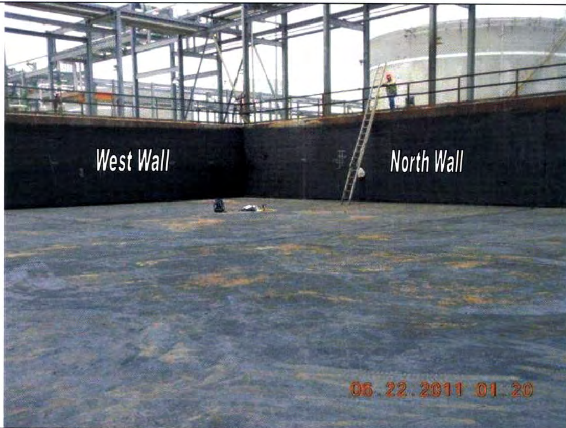
Photograph 9. Overview of the Southeast corner of the West Rain Basin.
