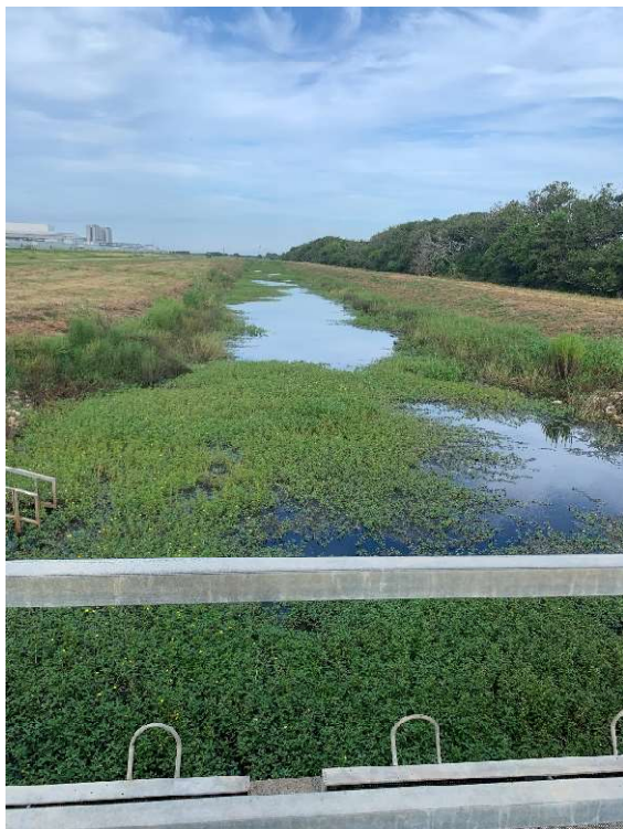
#2 Outfall 003 Up Stream (facing West) taken on 8/16/24
