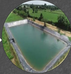
Storm Water Storage Pond
