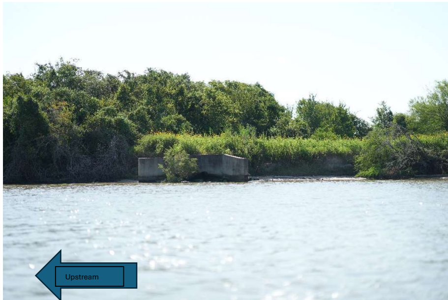
#1 Upstream of Outfall 001 (facing East) taken on 8/17/24
