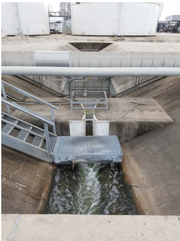
Photo 5. Outfall 004 at Parshall flume.
