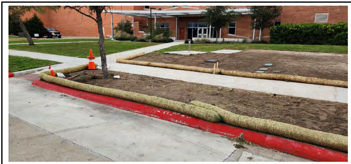
DMC Ground crews installed BMPs provided by EHS Office in an area disturbed by underground sprinkler repairs.
