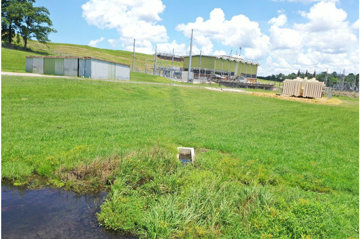
Photo 2: Proposed Outfall 004 point of discharge looking upstream
