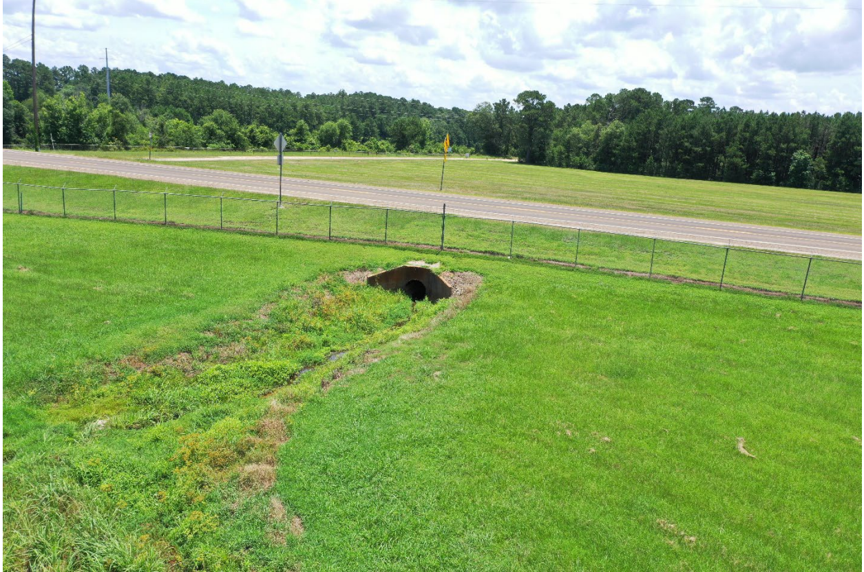
Photo 3: Proposed Outfall 004 point of discharge looking downstream
