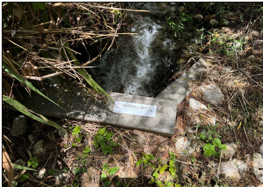
Photo 1 - View of Outfall 001
