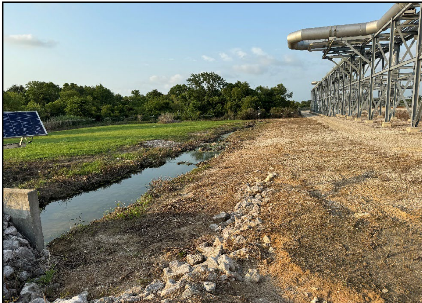
Photo 6 - View of Drainage Ditch Upstream of Outfall 002
