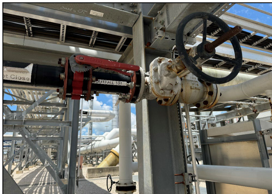
Photo 8 - View of Outfall 101
