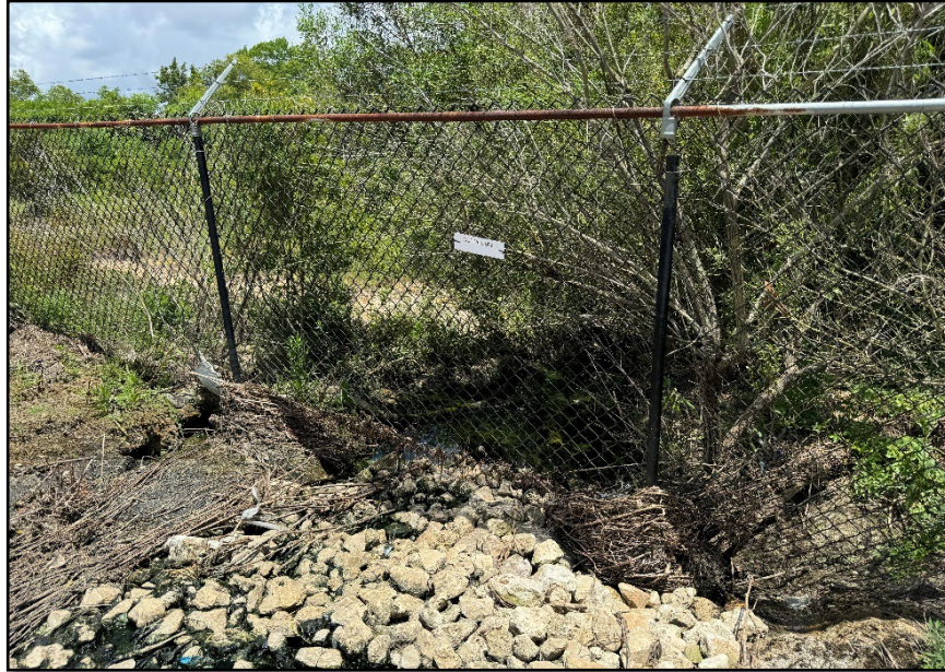
Photo 5 - View of Outfall 002
