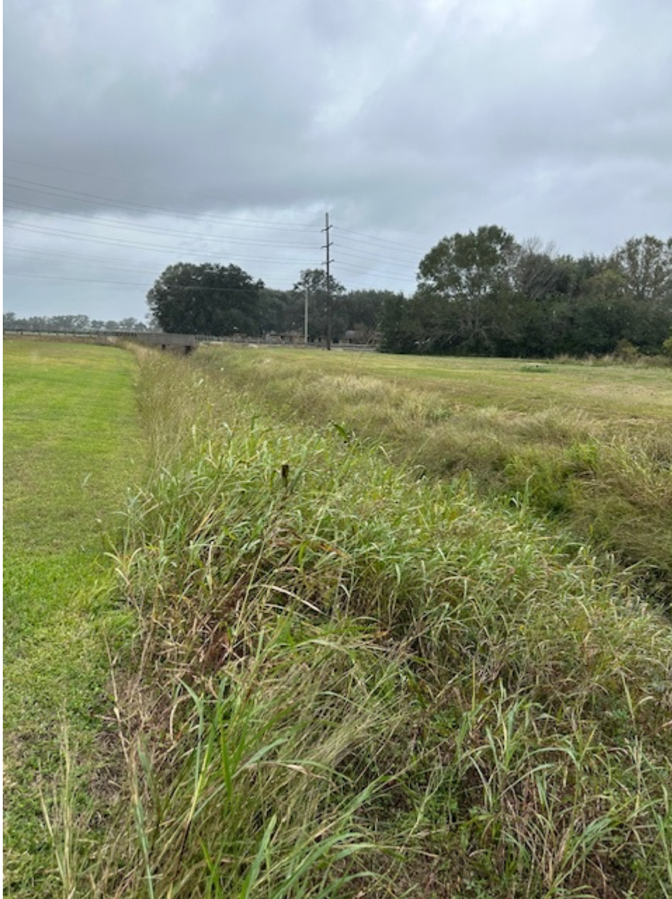
Photo 3 - Cow Island Bayou runs south after Hwy 90 for a short distance then turns east and runs along the south side of Raywood, TX. This photo is taken near the Precinct #1 Building almost 1-mile from the outfall discharge
