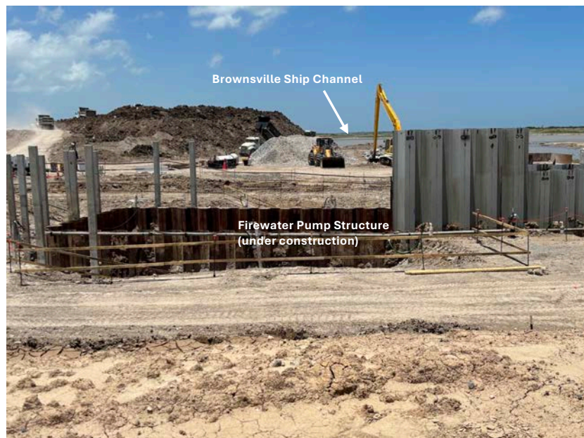
Photo 7 – Seawater Firewater Pump Structure (Outfall 004)
