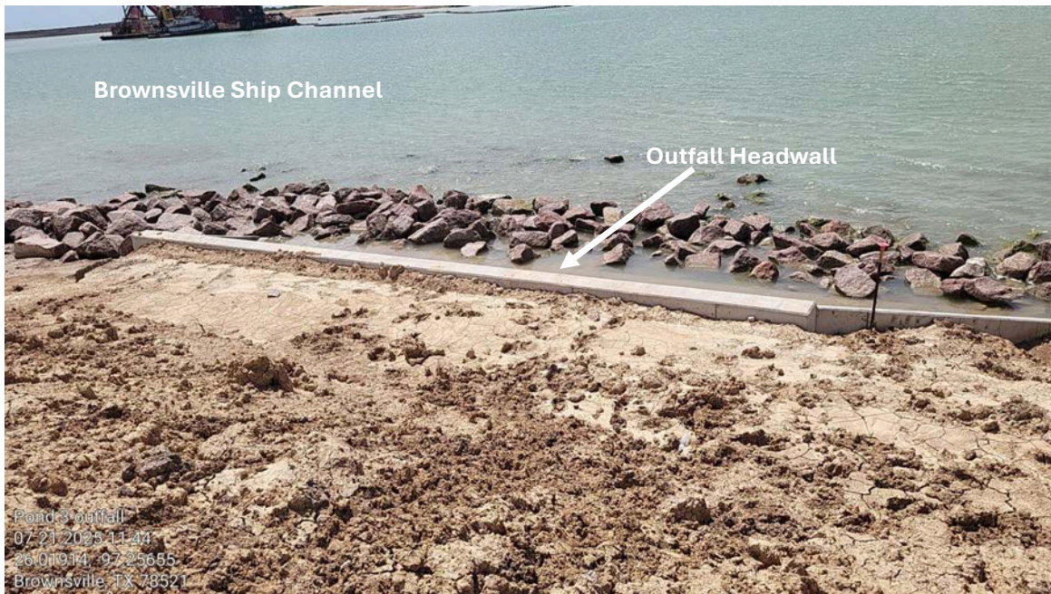
Photo 6 – Outfall 003 Headwall Structure
