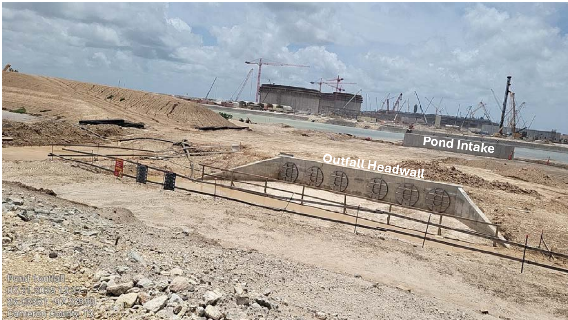
Photo 2 – Outfall 001 Headwall and Intake Structure
