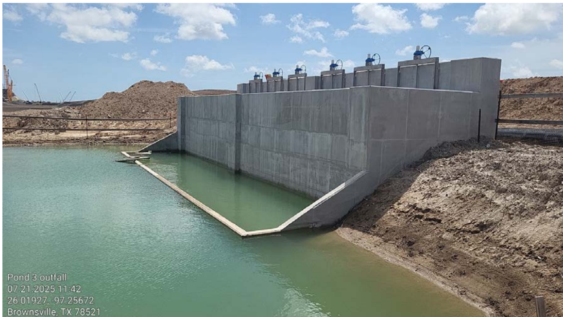
Photo 5 – Pond 3 Intake Structure
